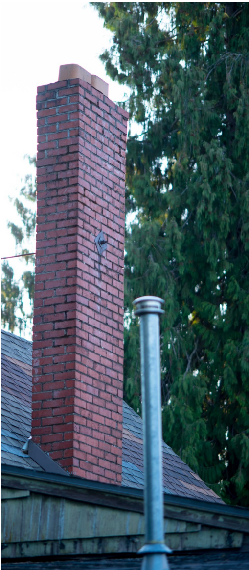
Figure 21: Chimney View At Back Looking Northeast
