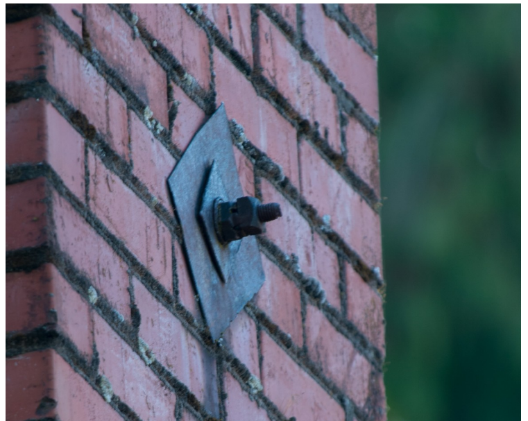
Figure 22: Chimney Brace Plate Detail
