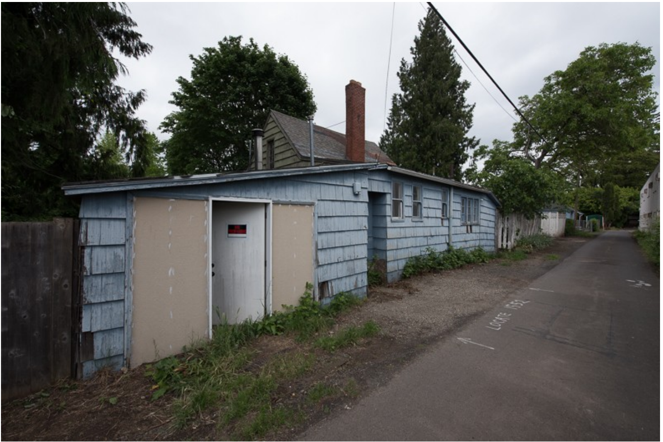
Figure 11: Garage Door Infill as of May 27, 2019
