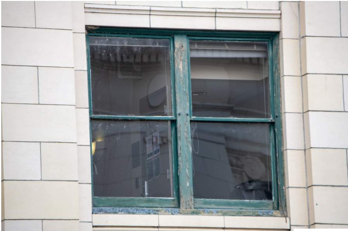
Figure 12 – Window on south elevation
