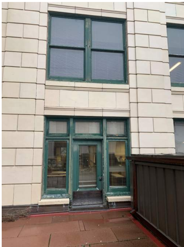
Figure 18- Wood door at light court on the South elevation
