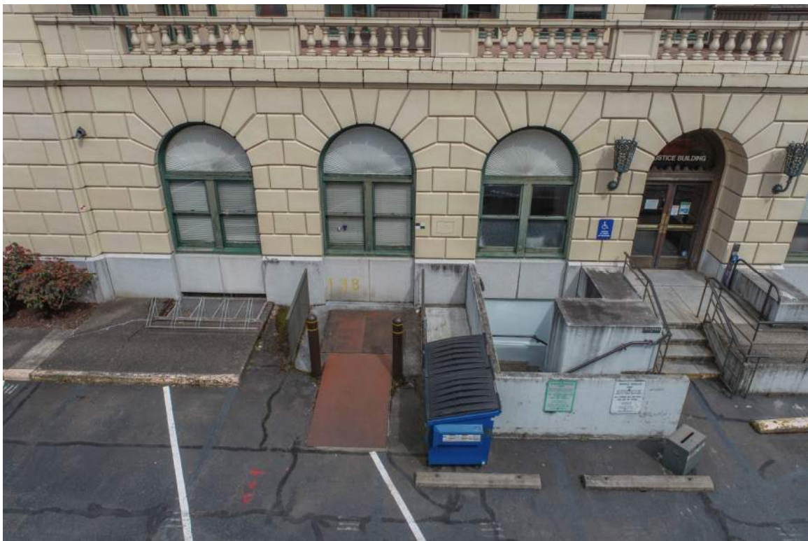
Figure 16 - Aerial view of sidewalk lift on south elevation
