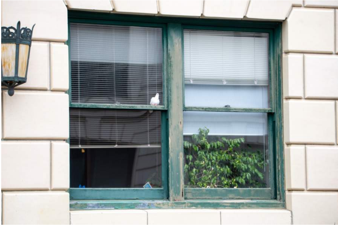
Figure 11 – Window on south elevation
