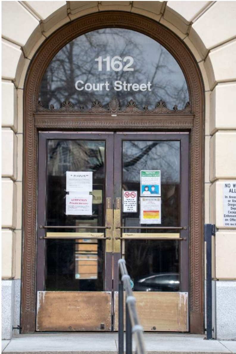
Figure 18 – Entry doors north facade
