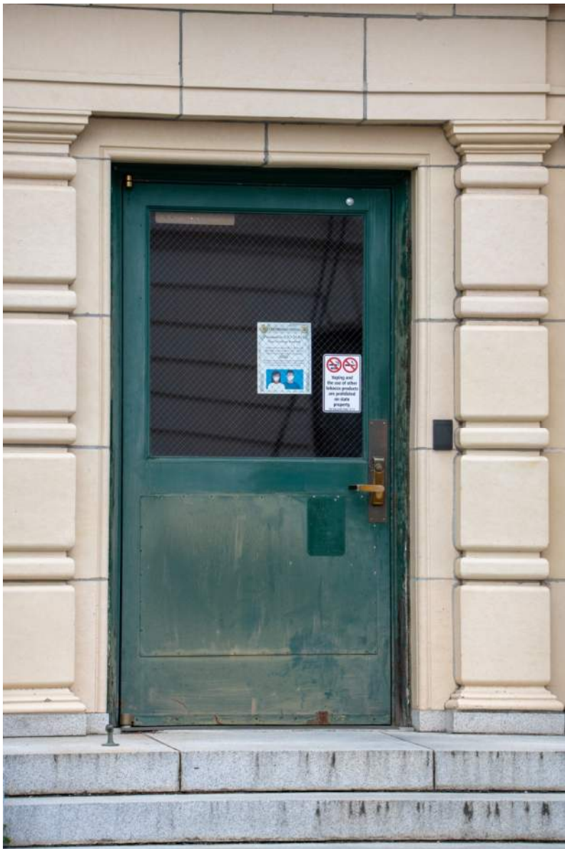
Figure 14 - Metal door on south elevation
