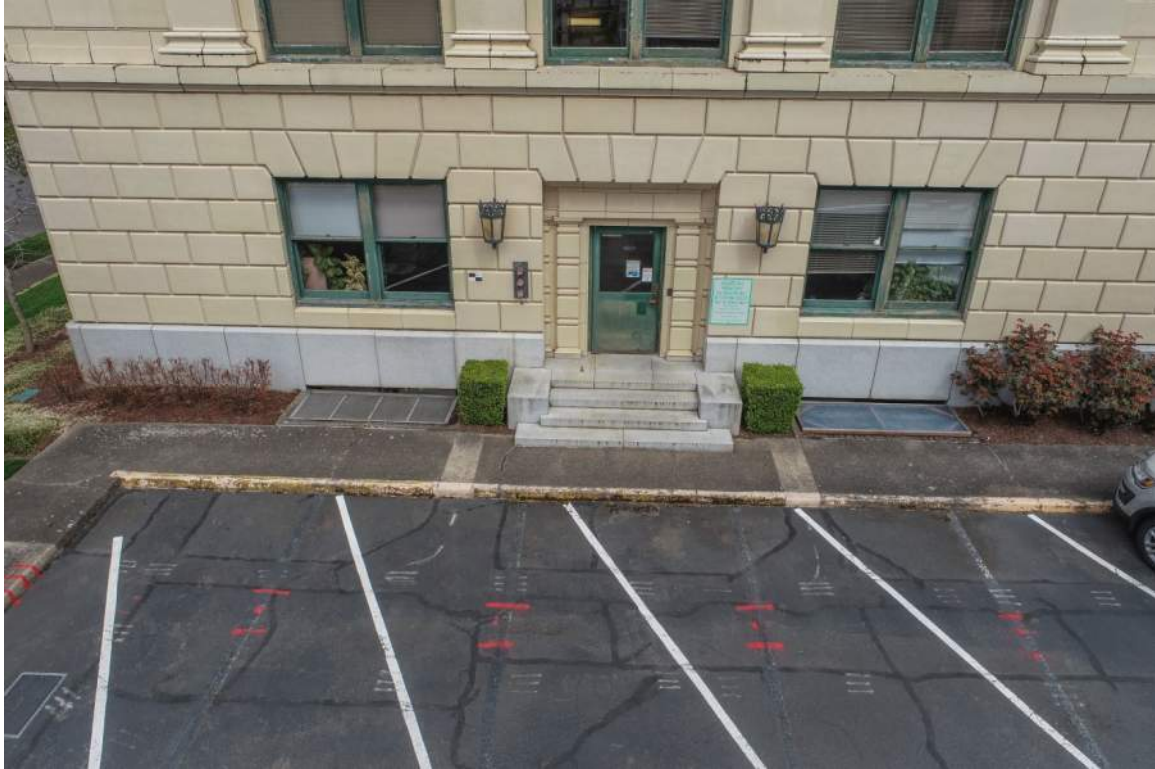
Figure 15 - Aerial review of south elevation and metal door
