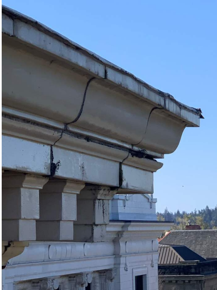
Figure 8 - Terracotta - Existing Conditions - Cornice
