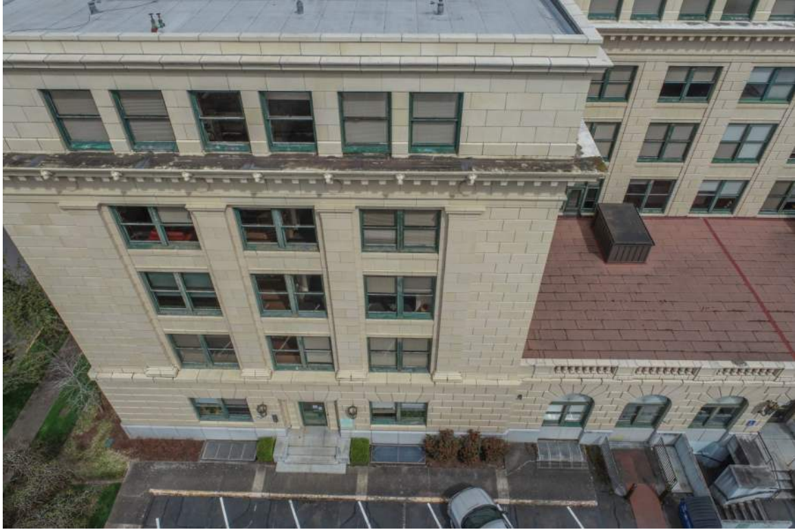
Figure 9 - Justice Building aerial view of cornice
