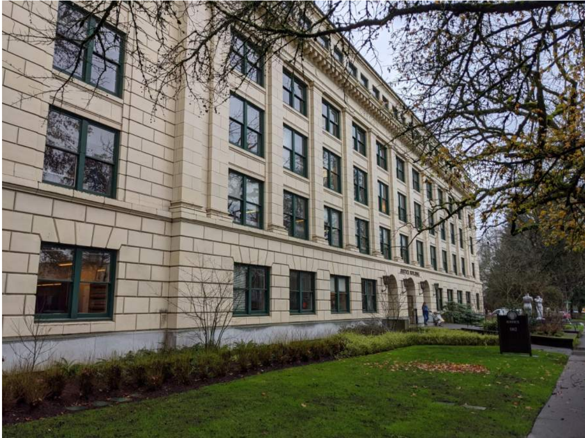
Figure 1- Justice Building North Elevation
