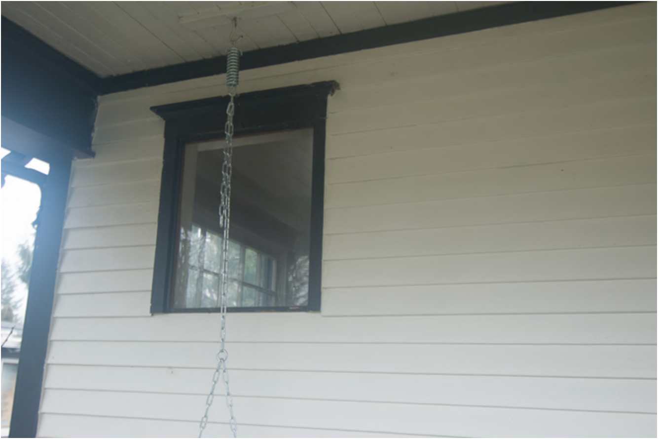
Illustration 23: Current Front Porch Window (February 9, 2019) – Replaced after 1970 with Plexiglass fixed window,
