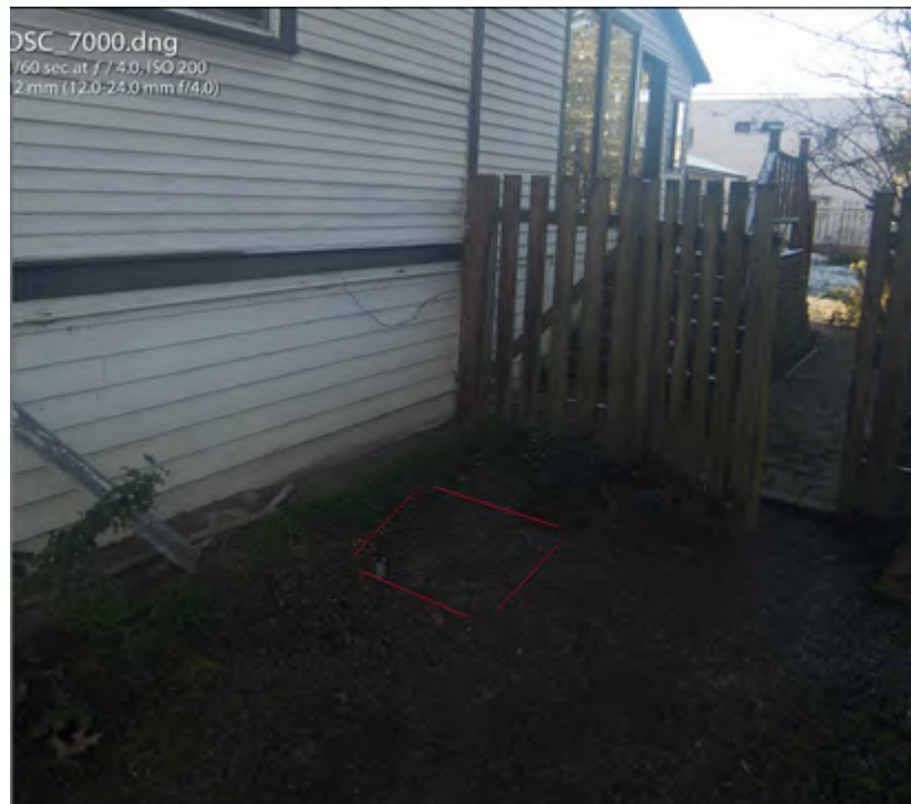
Illustration 16: Air Conditioning Condensor Location
