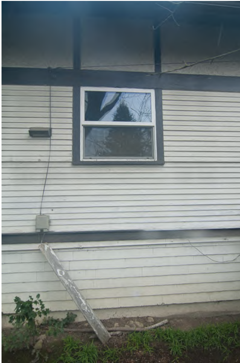
Illustration 20: Kitchen Vinyl Window On Western Facade
