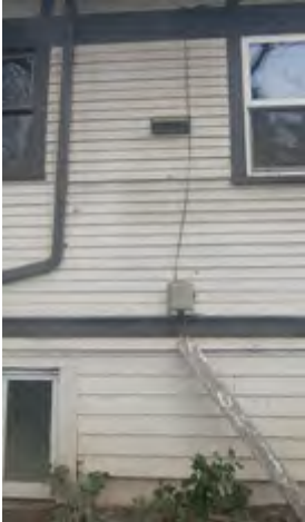
Illustration 12: Existing Kitchen Vent On West Wall
