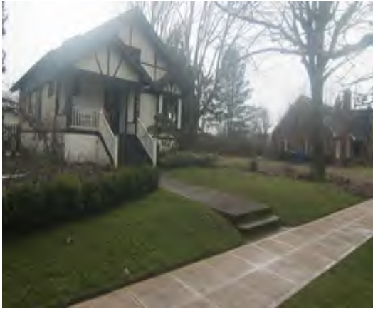
Illustration 18: 1566 Court Street NE - stairs from sidewalk
