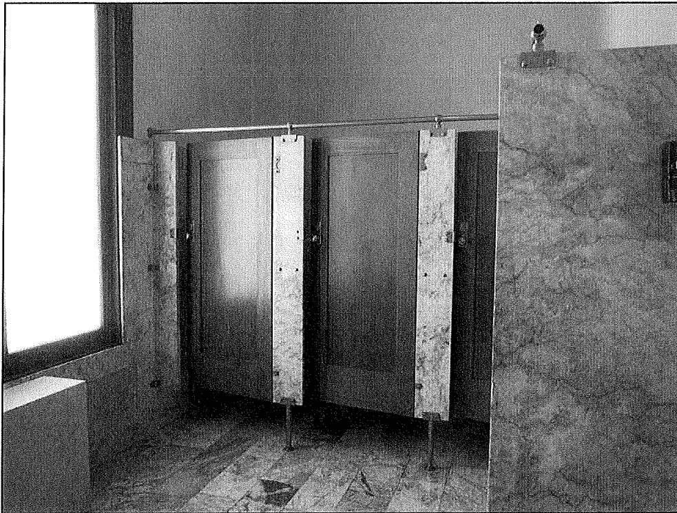
Photo 9 of 14: The third floor men's restroom with marble partitions and mahogany doors, typical of all original restrooms. Camera facing east.
