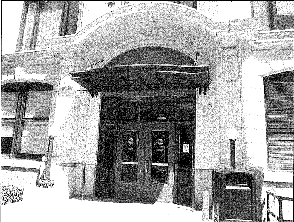
Photo 4 of 14: Primary south (public) entrance, camera facing north.
