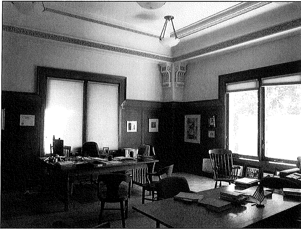
Photo 13 of 14: The original Chief Justice's office in the southeast corner of the third floor. Camera facing southeast.
