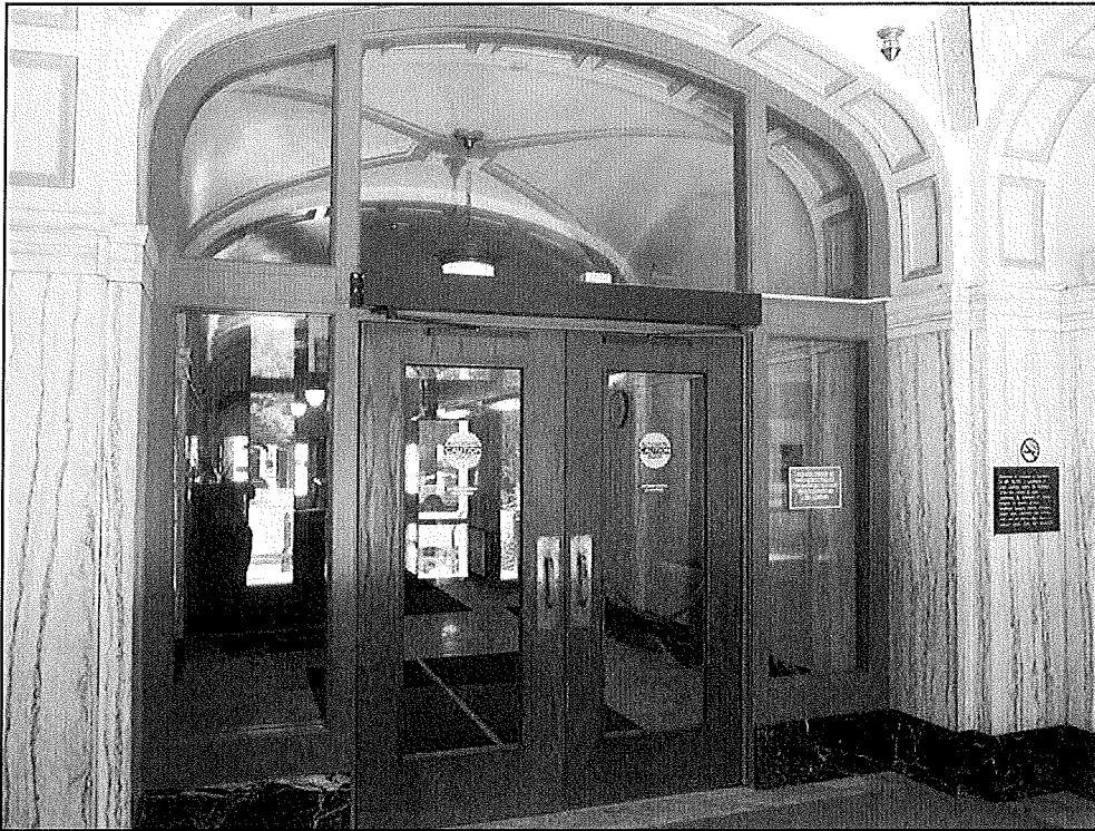
Photo 5 of 14: South entrance vestibule leading into the first floor corridor. Camera facing north.
