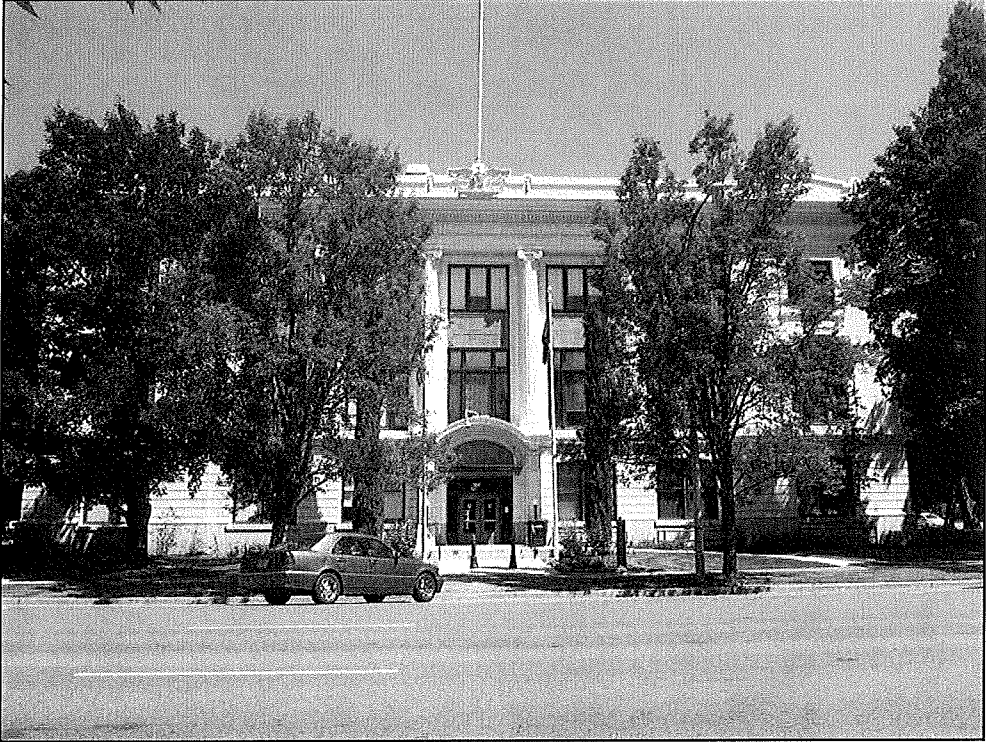
Photo 1 of 14: South elevation from State Street, camera facing north.
