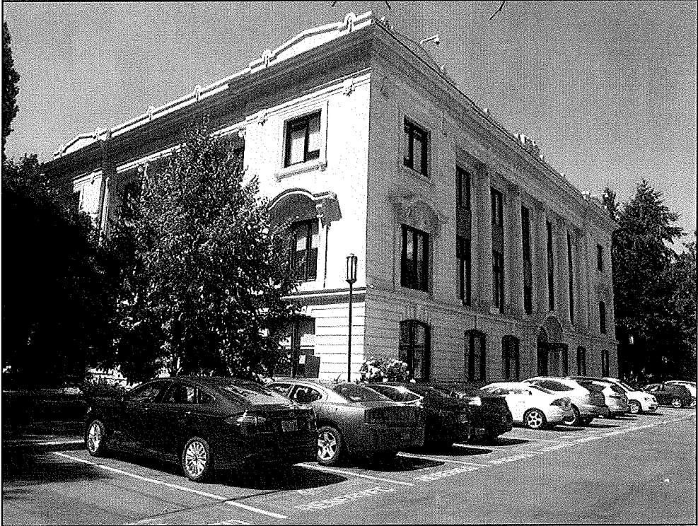
Photo 2 of 14: Northeast corner from 12 th Street Northeast, camera facing southwest.
