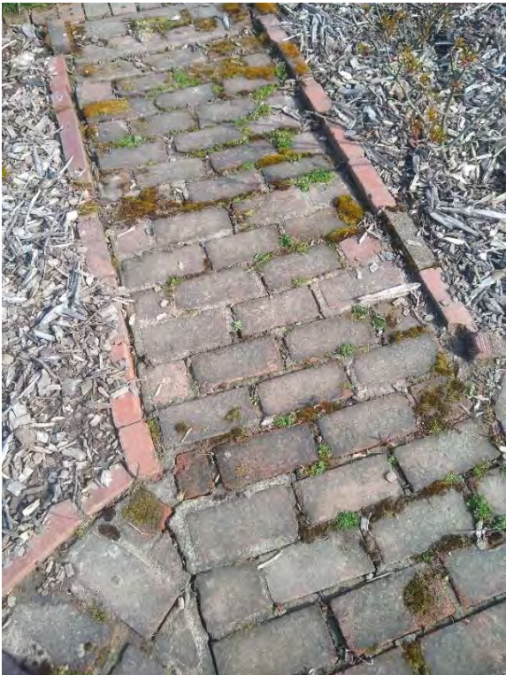
Closeups of the brickwork.
