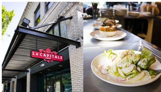
La Capitale Brasserie, located at the corner of State and High Streets, is part of Downtown’s successful “restaurant row.”
