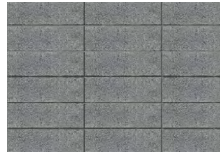
FURNISHING/PLANTING ZONE, DARK CONCRETE, 1'X3' SCORING GRID
