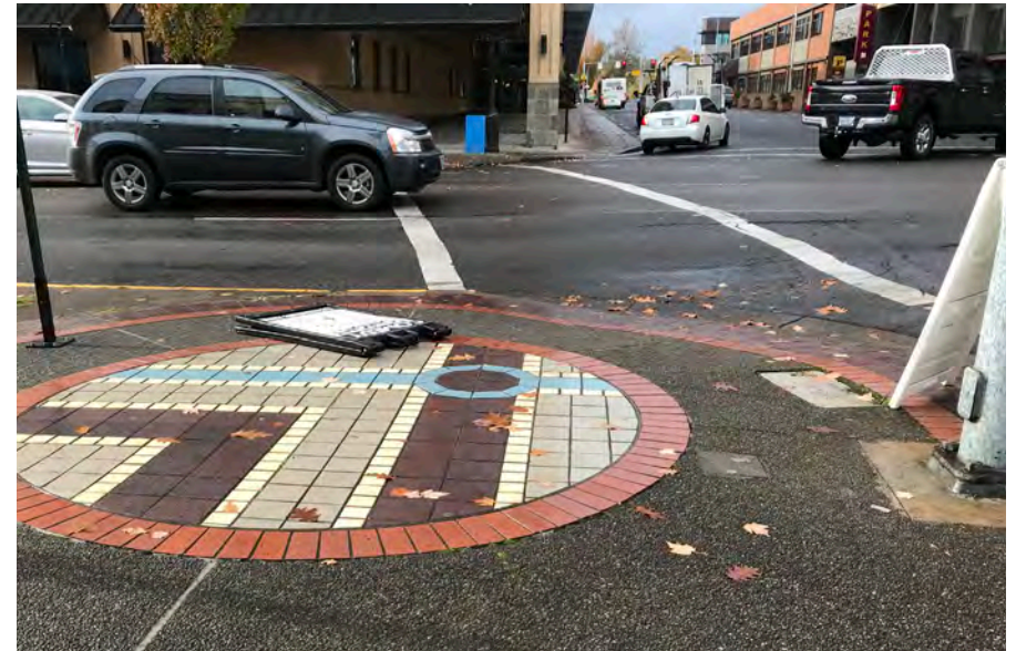
Remnants of previous streetscape project
