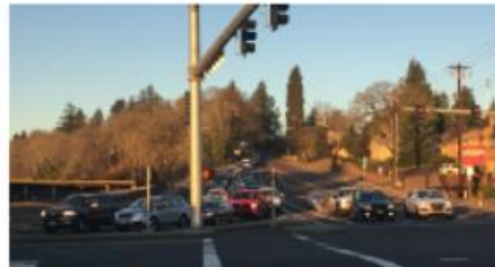
Wallace Rd. at Glen Creek Rd.
