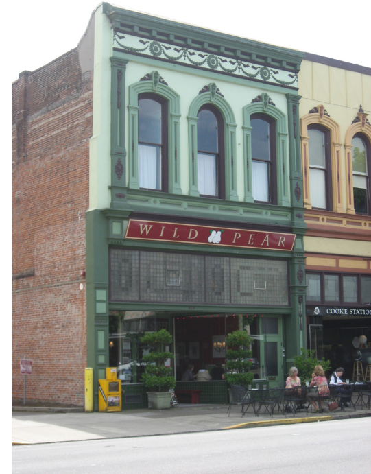
The building that houses Wild Pear, an independent restaurant, is an example of a URA toolbox investment and the historic character of the downtown core.
