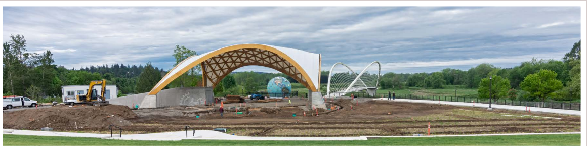
Gerry Frank | Salem Rotary Amphitheater under construction (2021)
