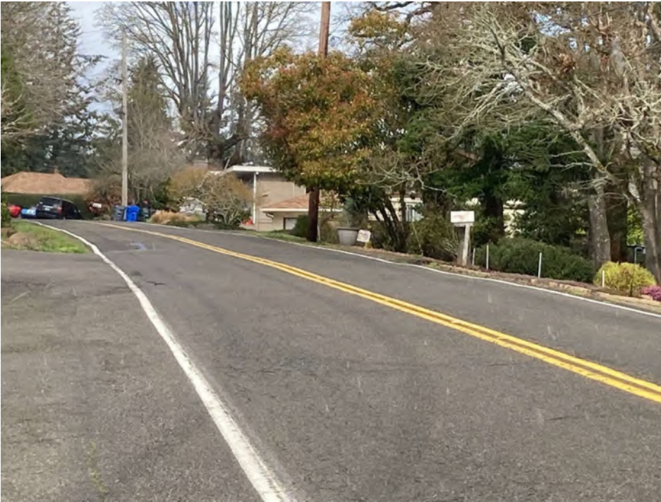
Existing narrow cross section on College Drive (driveway to right is one providing access to subject property)
