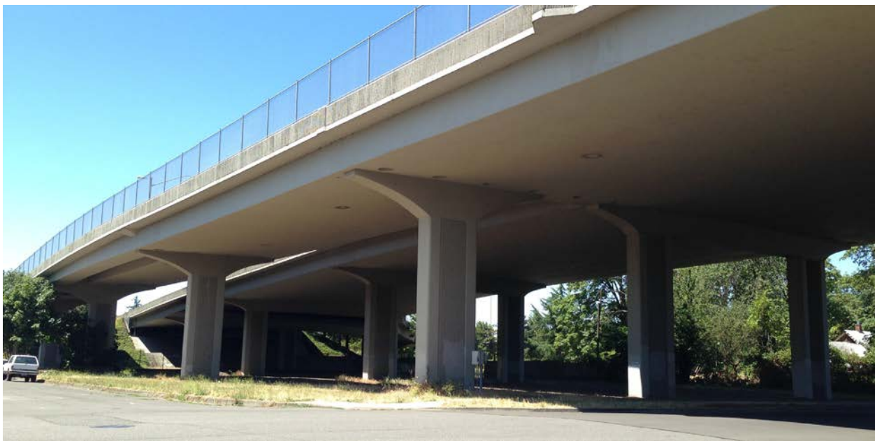
Figure 30 Vacant area under Mission Street bridge in SESNA
