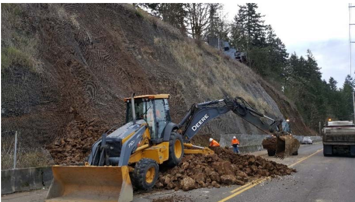
January 2018: Backhoe removing slide debris
