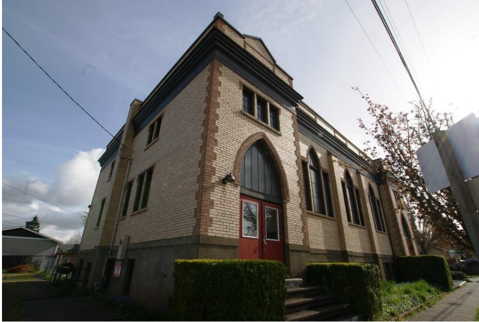
Photo 3 of 53 (Cottage_905_NE_03) South and west elevations, view northeast.
