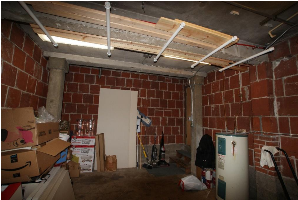
Photo 32 of 53 (Cottage_905_NE_32) Basement utility room, view east.
