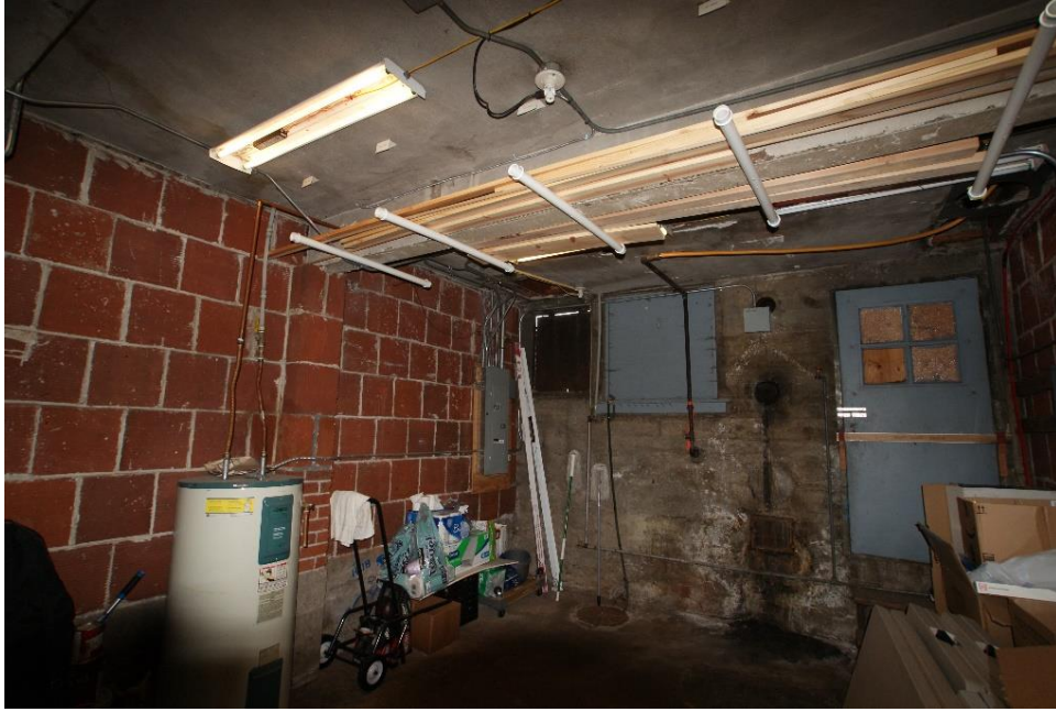
Photo 31 of 53 (Cottage_905_NE_31) Basement utility room, view northwest.
