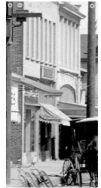
HISTORIC SOUTH ELEVATION
