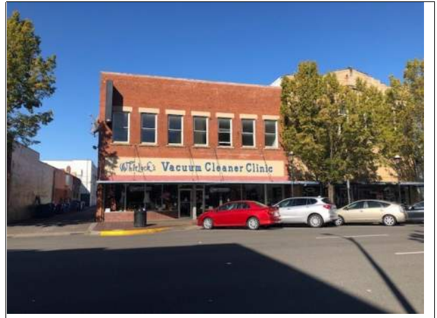
D'Arcy Building Looking North
