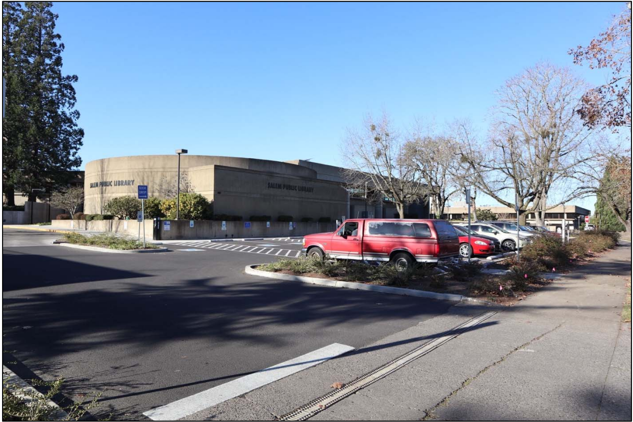
Photo 31 of 40. Public Library south and east elevations, looking northwest.
