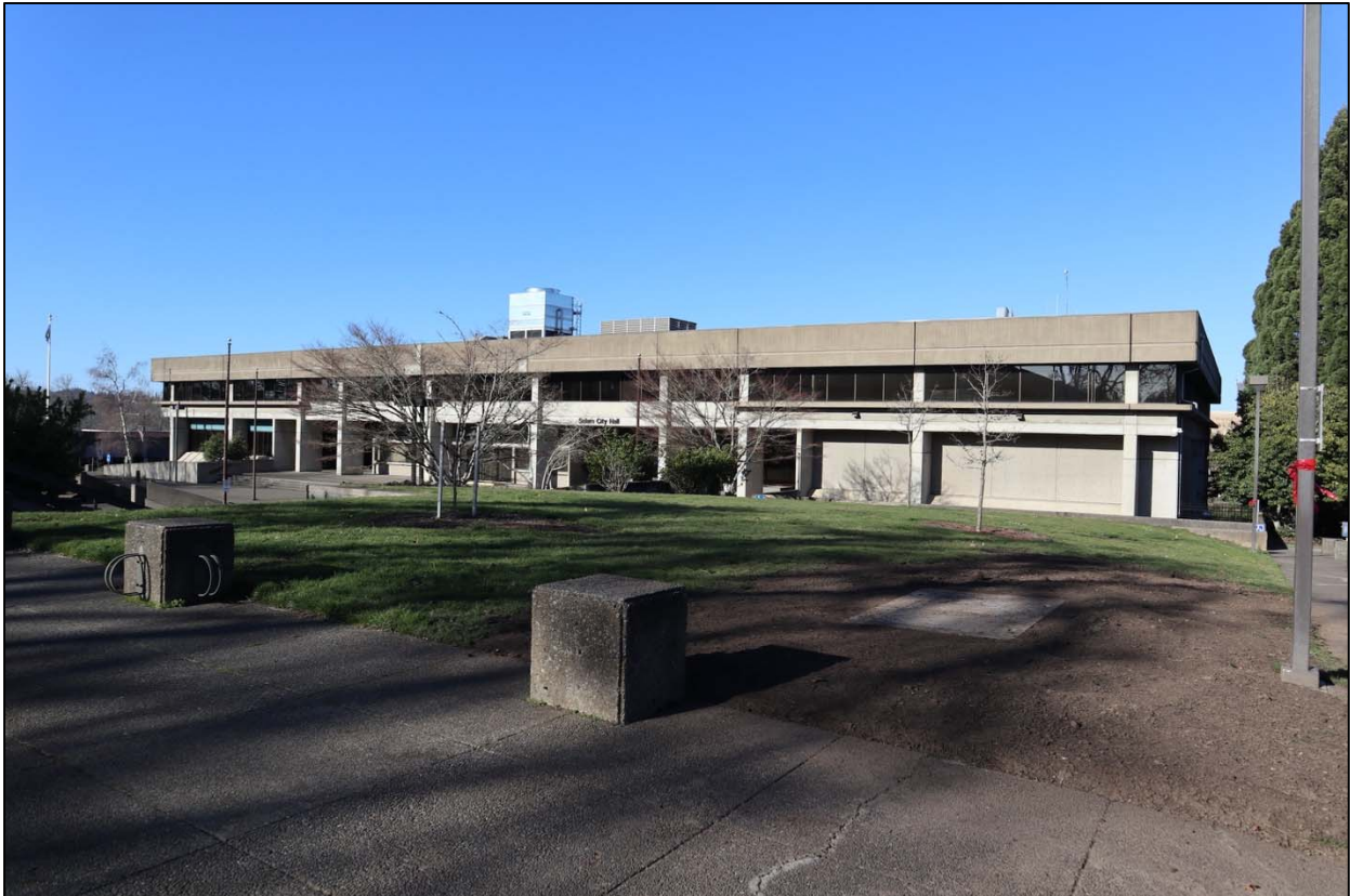
Photo 18 of 40. City Hall south elevation, looking northwest.
