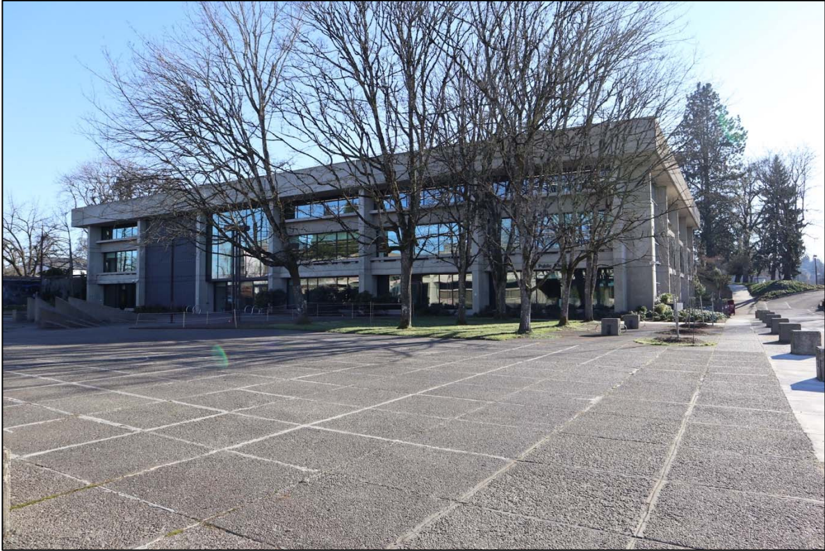
Photo 29 of 40. Public Library north elevation, looking southeast.
