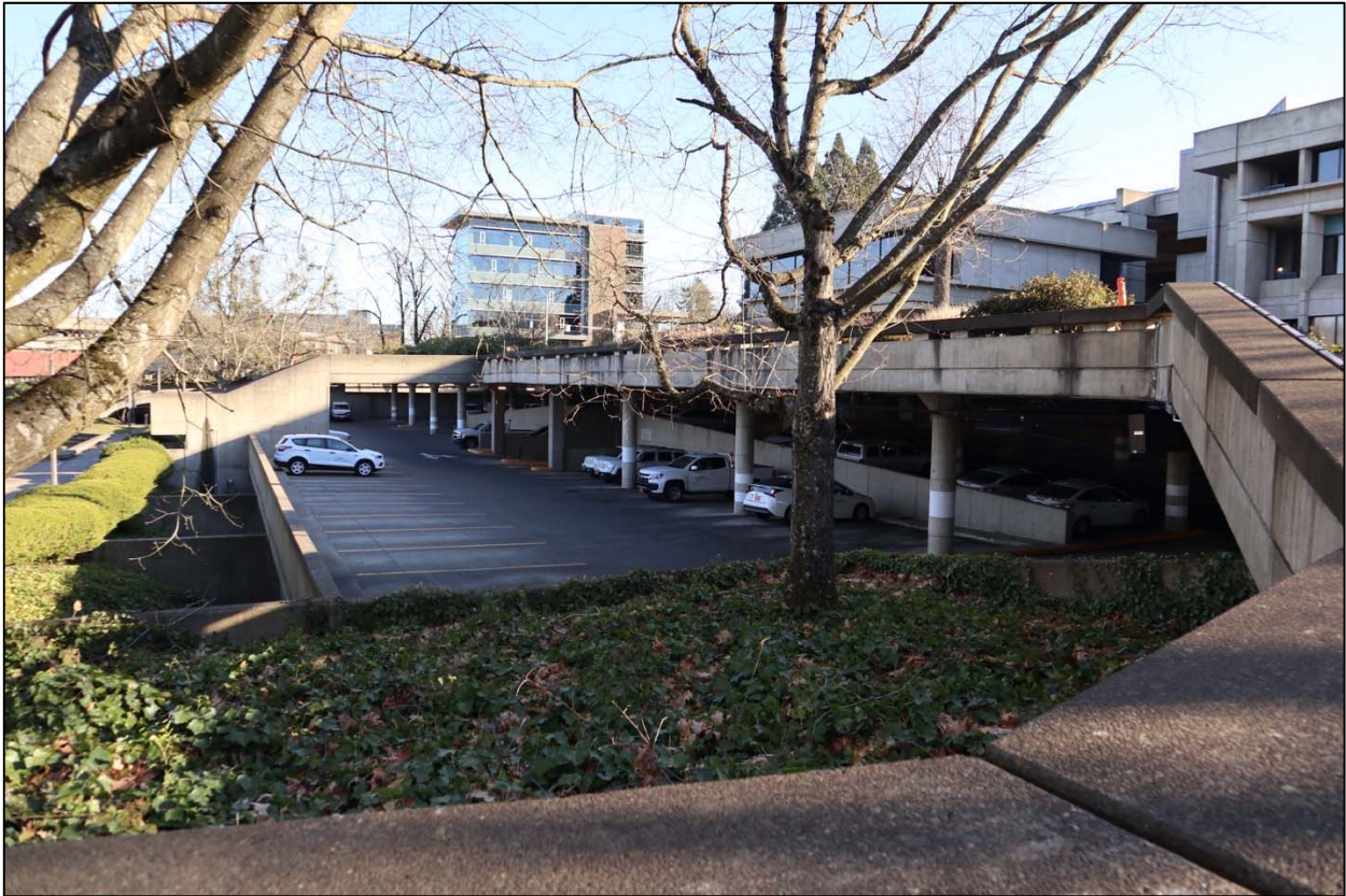
Photo 11 of 40. City Hall Parking Garage, looking east.
