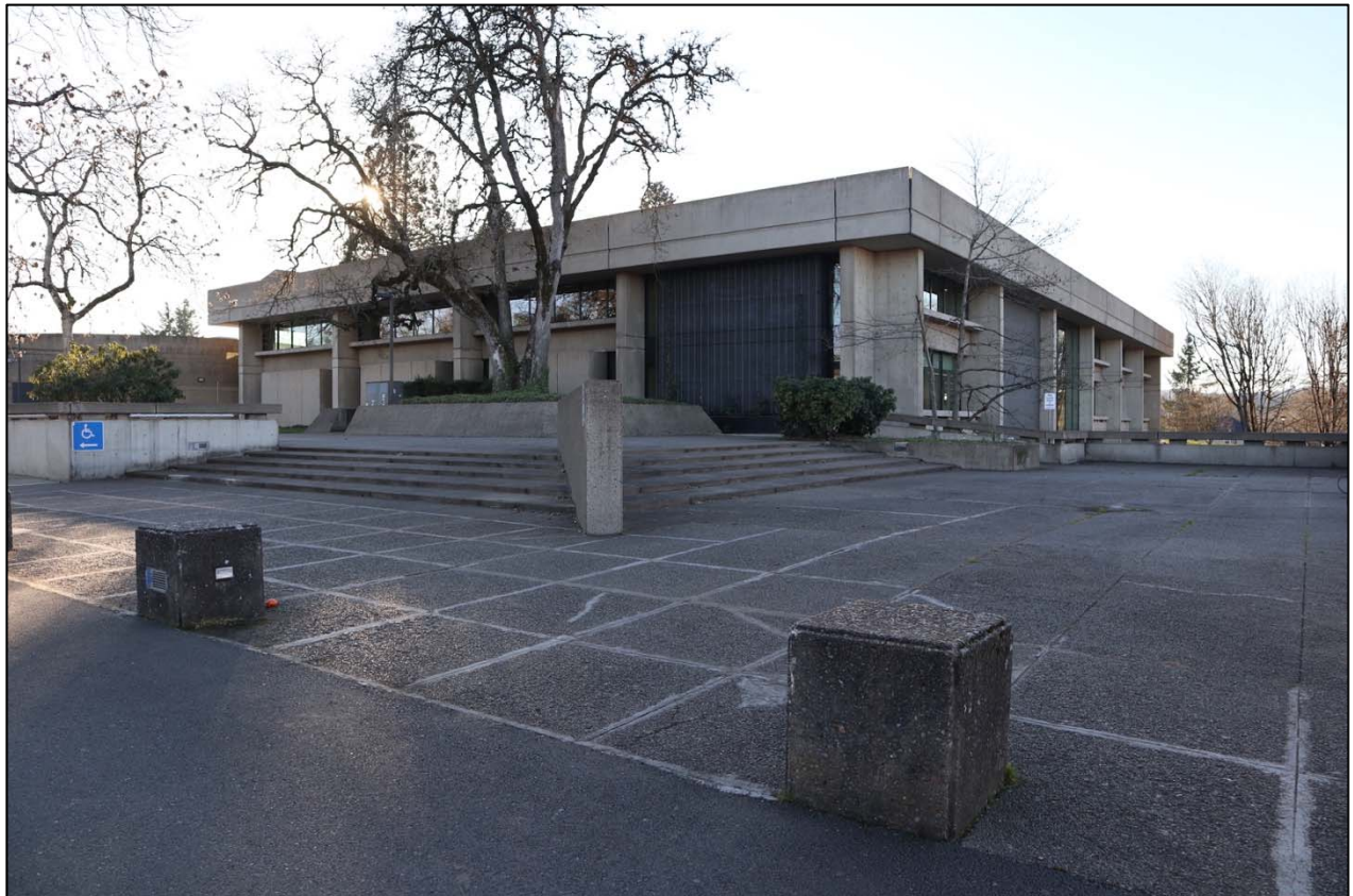
Photo 32 of 40. Public Library north and east elevations, looking southeast.
