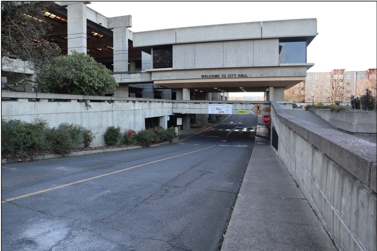
Photo 14 of 40. City Hall Council Chambers, looking west
