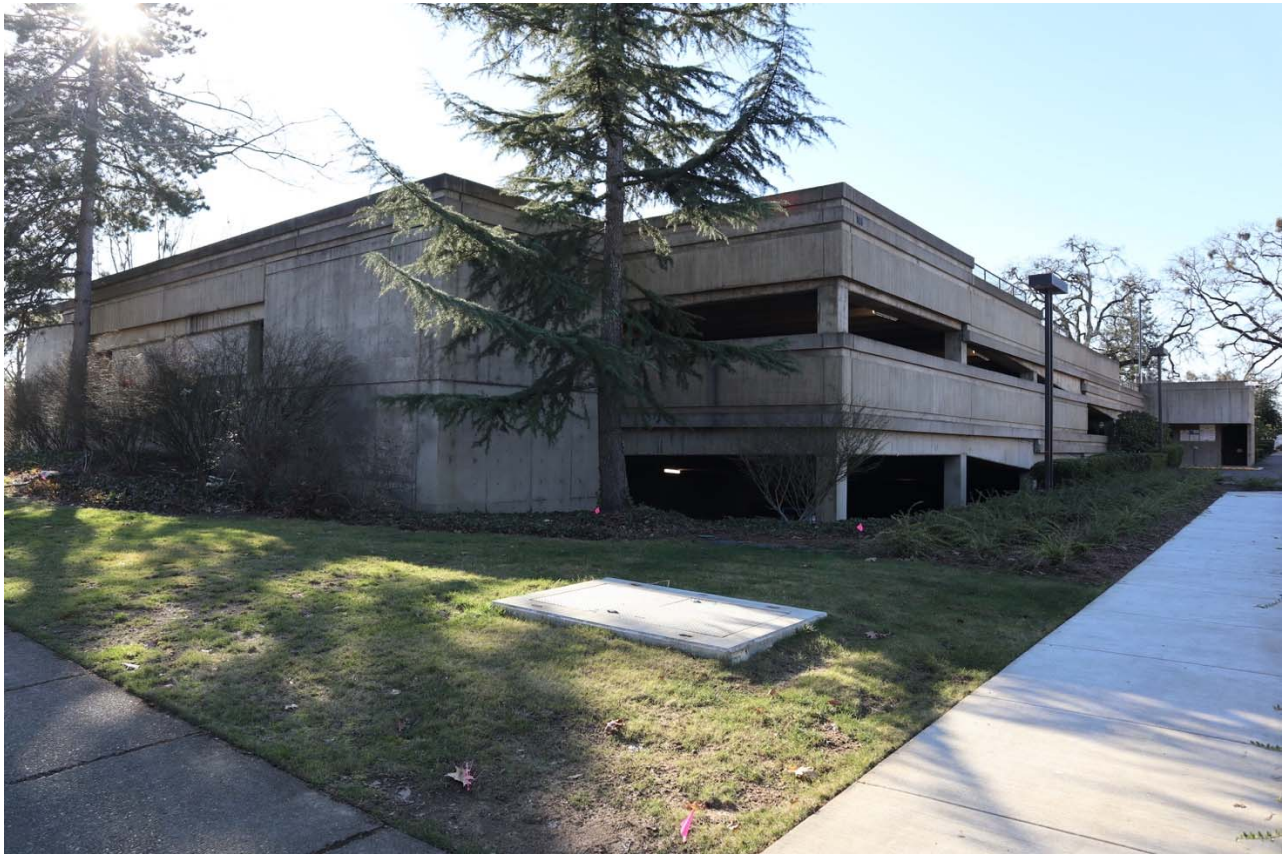
Photo 33 of 40. Public Library Parking garage, looking southwest.
