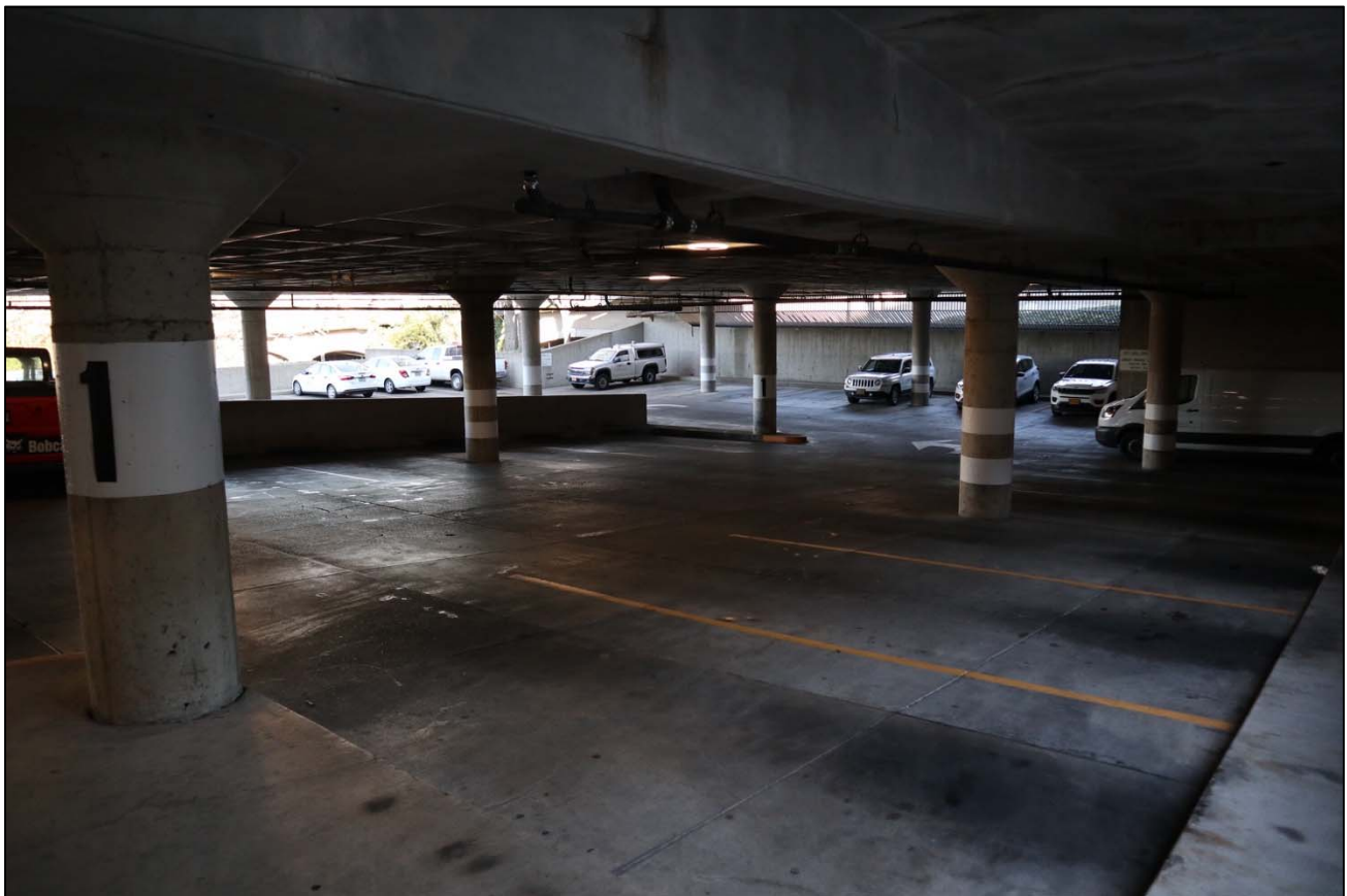
Photo 12 of 40. City Hall Parking Garage, looking northeast.
