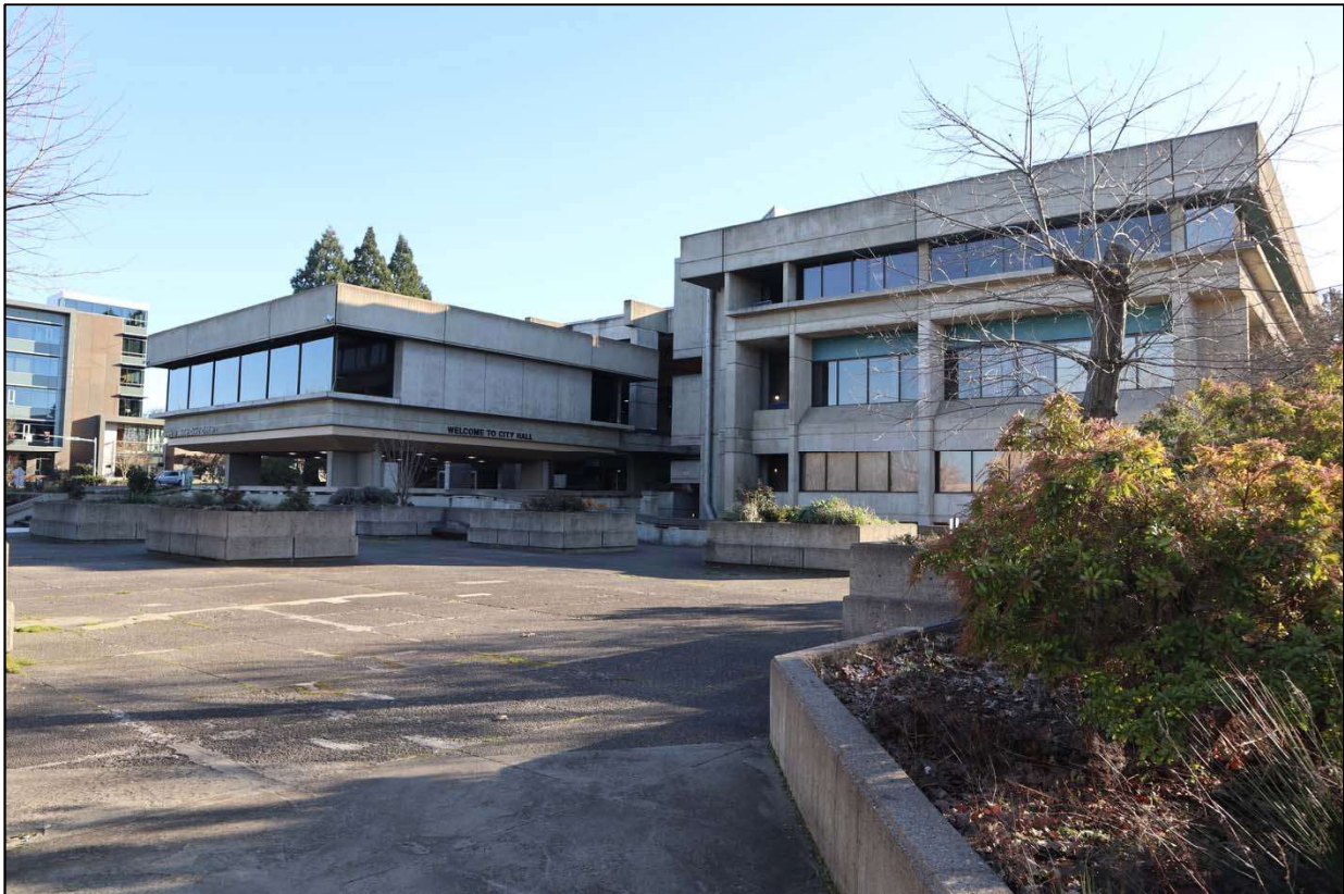
Photo 16 of 40. City Hall north elevation west bay, looking southeast.
