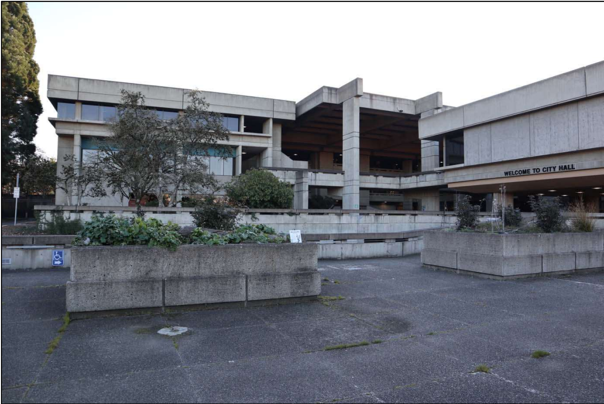
Photo 15 of 40. City Hall north elevation east bay, looking south.
