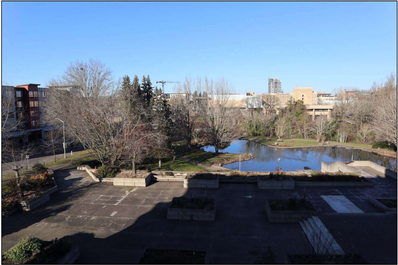
Photo 5 of 40. Overview of the Salem Civic Center, looking north.
