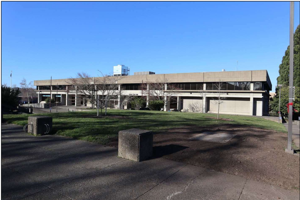
Photo 18 of 40. City Hall south elevation, looking northwest.
