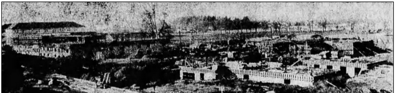
Yaquina Hall under construction, 1948.
