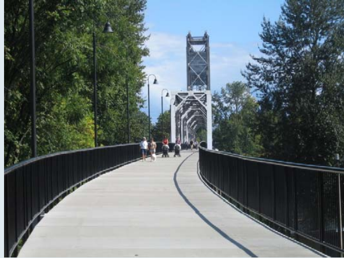
Union Street Railroad Pedestrian and Bicycle Trail
