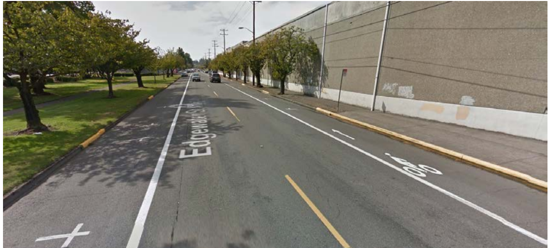
Large blank walls along the west end of Edgewater create a challenging environment for bicycles and pedestrians.
