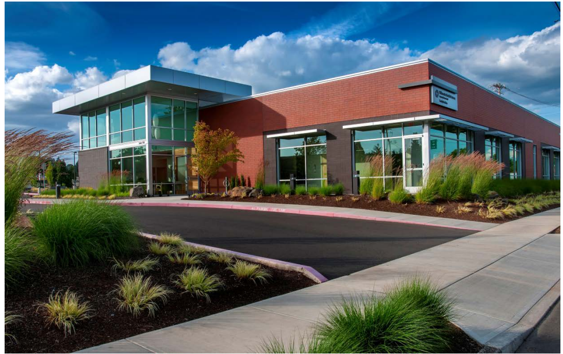
Several new medical offices and clinics have located in the Main Street Area along 2 nd Street.
