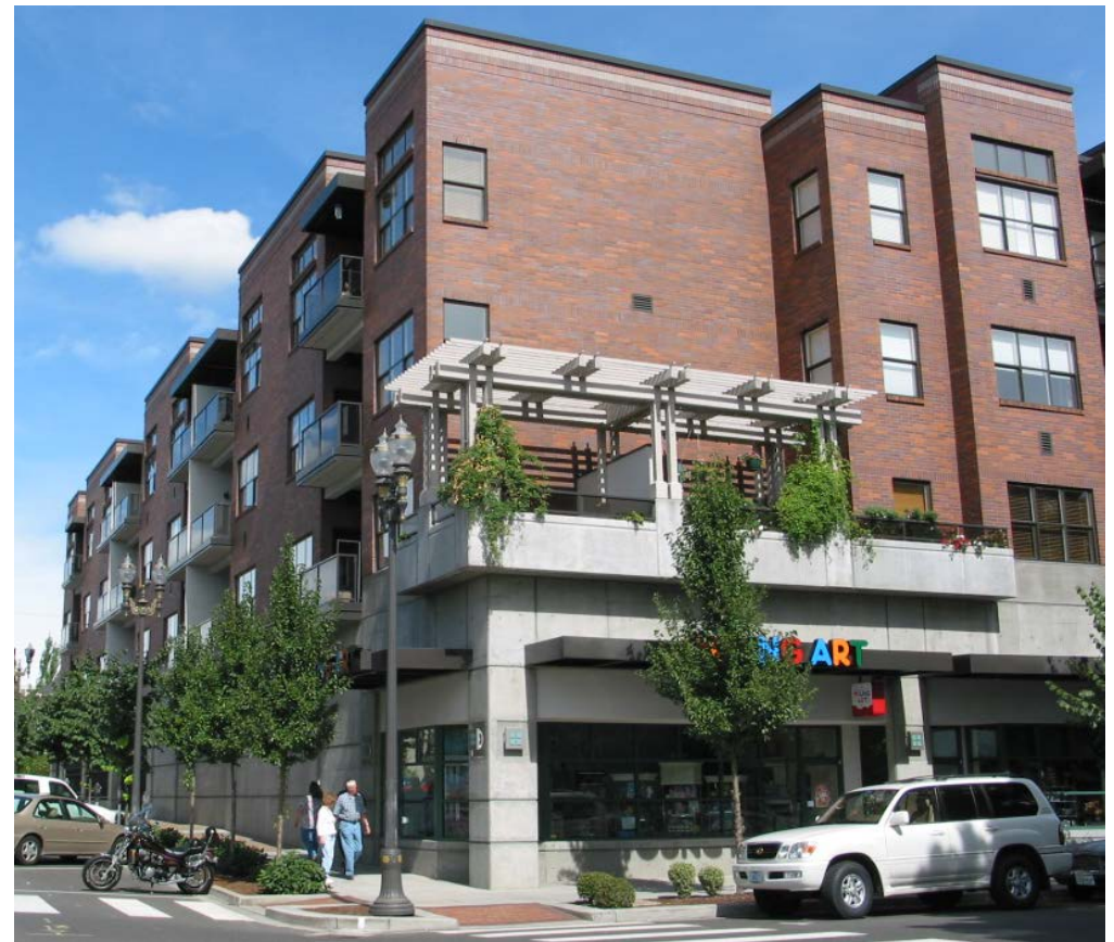
Example of mixed-use development potentially suitable for West Salem Town Center.
