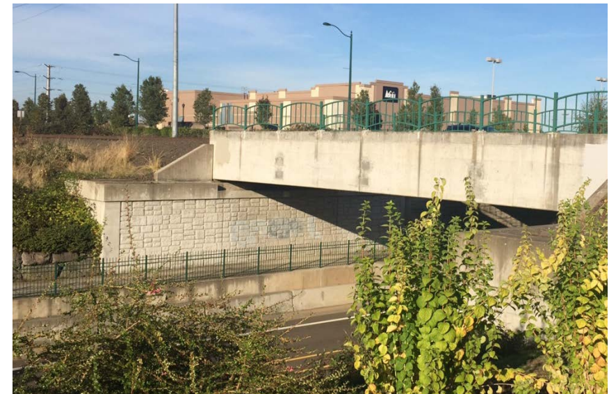
Example of elevated multi-use path along an underpass on Keizer Station Blvd, crossing under Stadium Dr. in Keizer.
