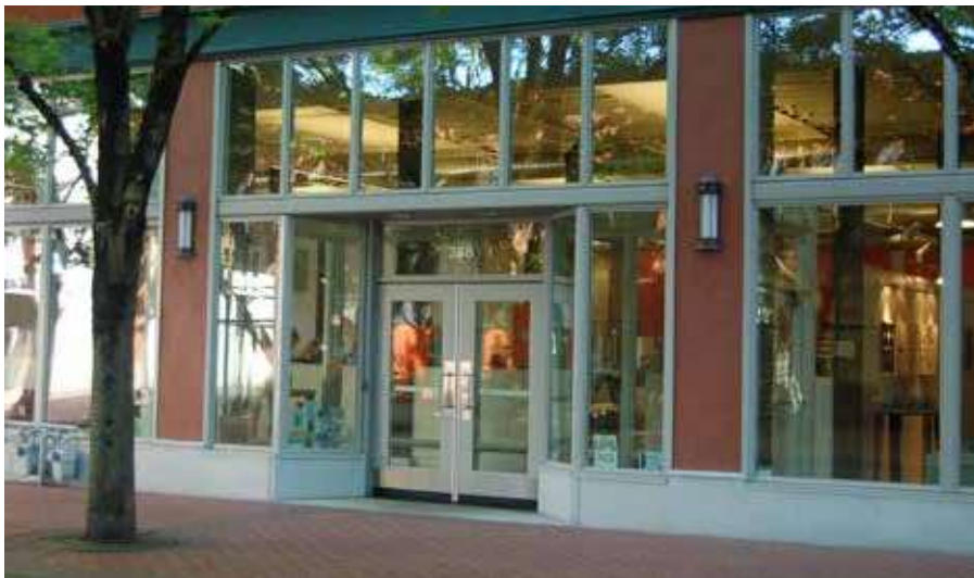
The new storefront system at the historic Minnesota Hotel building has a fine-grain level of detail.
