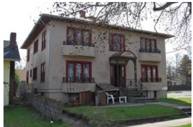
1710 CAPITOL ST NE, BUILT 1930
