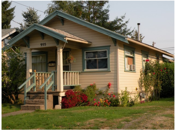
955 JEFFERSON ST NE (DEMOLISHED 2010 BECAUSE OF FIRE), BUILT 1922
