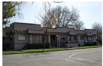
1000 CAPITOL ST NE, BUILT 1946
