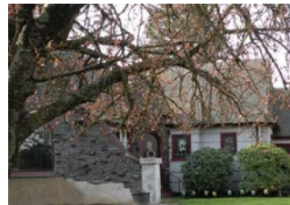
1170 NEBRASKA ST NE, BUILT 1935
