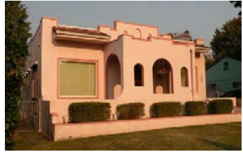
1265 SUMMER ST NE, BUILT 1925
