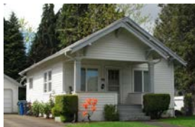
840 NORWAY ST NE, BUILT 1928
