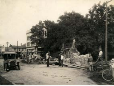
Construction of a street in Salem, Oregon. Taken 1912. Image courtesy of Willamette University Archives and Special Collections, Salem Eastern Oregon Photographs
