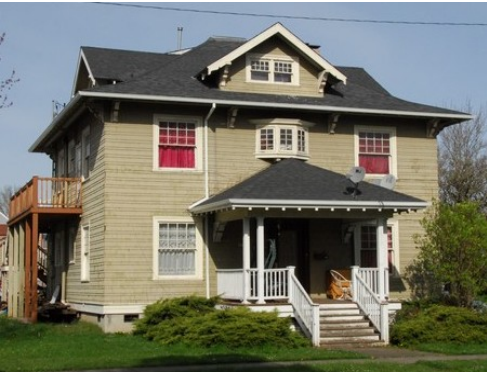
1075 CAPITOL ST NE, BUILT 1910
