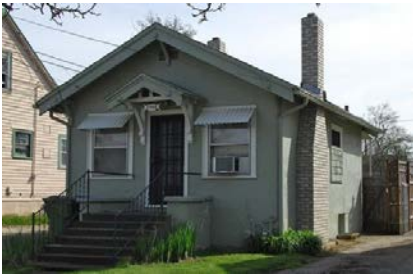
1740 CAPITOL ST NE, BUILT 1920
