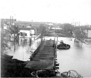
Photograph of the damage to the timber wagon bridge, looking north from Fry Hill in Salem, 1890. Photo courtesy of the Marion Co. Historical Society.
