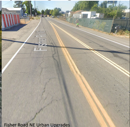
Fisher Road NE Urban Upgrades
