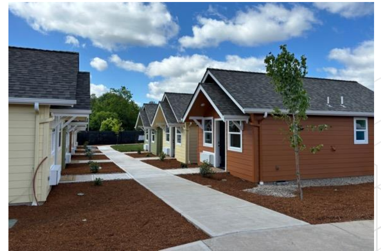
Housing Project Examples: Redwood Crossings, Salem Housing Authority; Cottage Clusters, United Way of Mid-Willamette Valley
