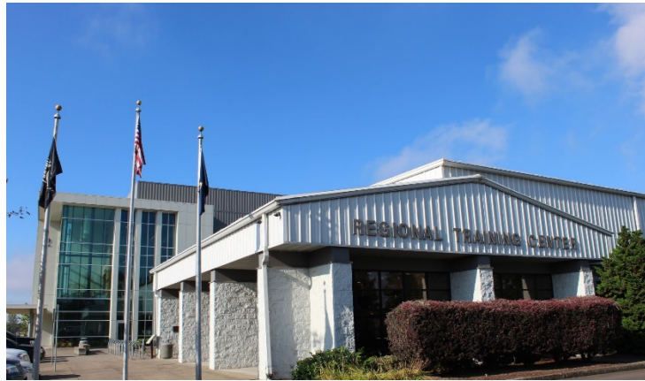
Brooklake Rd. NE west of intersection of Pueblo Ave. NE – Looking South
