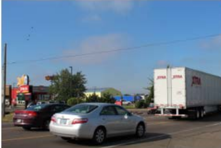
Brooklake Rd. NE – Directly West of I-5 Interchange – Looking South
