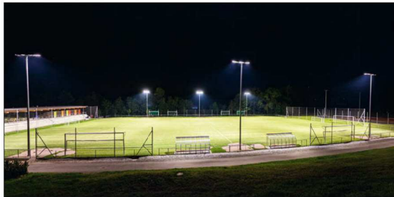
FIELD LIGHTING Product: Siteco '5XA77PFS3K' Fully Shielded Fixture 0% Upward Light Ratio Color: Black Masts and Fixtures Height: 80' See Exhibits for Lighting Distribution Plans.
