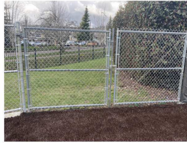
PERIMETER AND OUTFIELD FENCING AND GATES Metal Chainlink Fence Galvanized Finish Height(s): 8'-0", 6'-0", 3'-6" Black Vinyl Finish Height(s): 3'-6"
