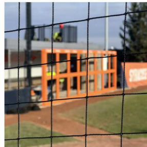
PROTECTIVE FIELD NETTING Light-weight fiber netting, 95% open-area Black Steel Posts Manufacturer: SportsField Specialties Color: Black Height: 40'-0" for pedestrian and adjacent property protection.
