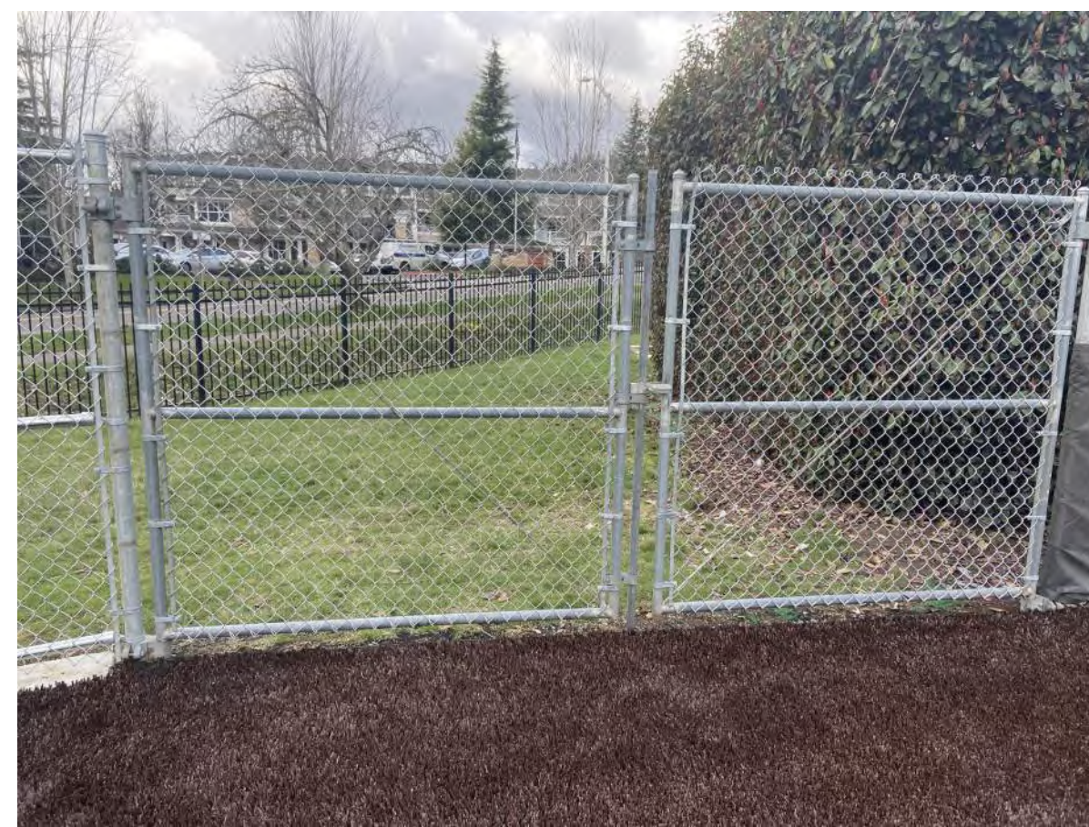
PERIMETER AND OUTFIELD FENCING AND GATES Metal Chainlink Fence Galvanized Finish Height(s): 8'-0", 6'-0", 3'-6" Black Vinyl Finsh Height(s): 3'-6"
