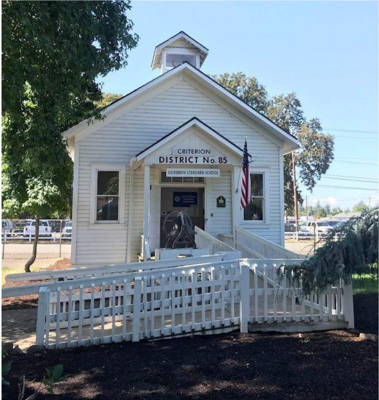
Image 10: East elevation of Criterion Schoolhouse. Source: Kirsten Straus 2023.
