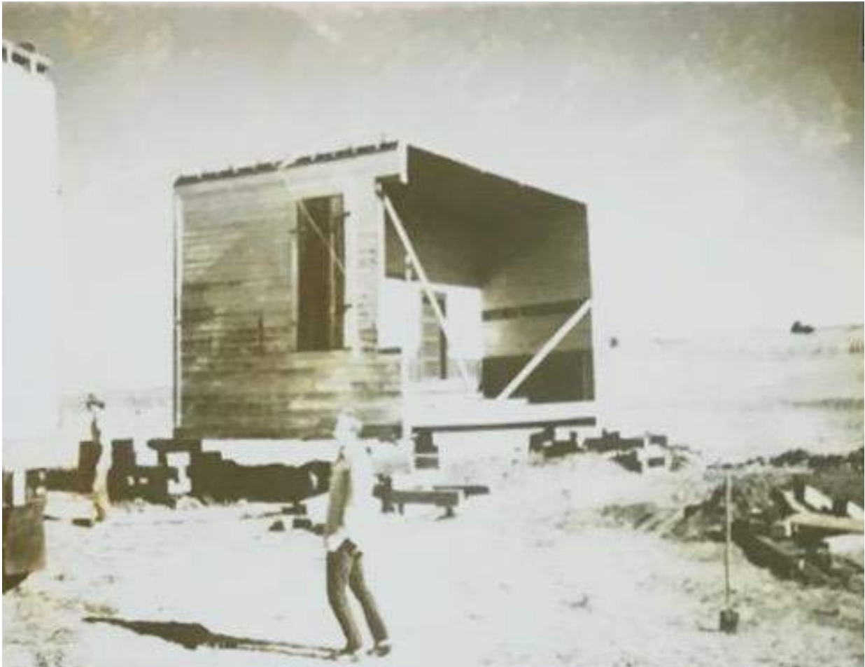
Image 6: Image of Criterion Schoolhouse cut in half and braced for transport. Source: Criterion Schoolhouse Committee (Oregon State Fair Foundation) image collection.
