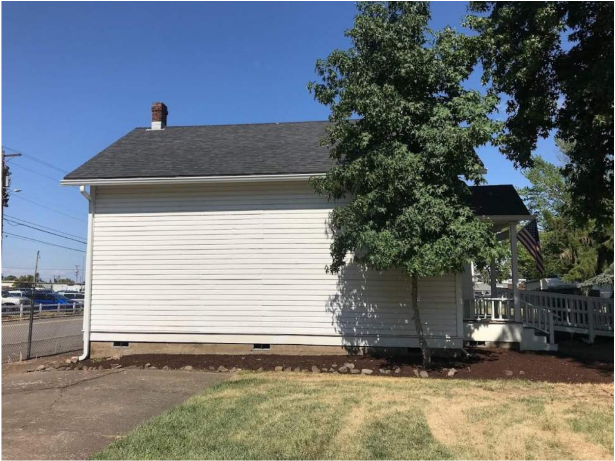
Image 13: South elevation of Criterion Schoolhouse. Source: Kirsten Straus 2023.
