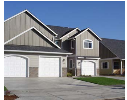
Built in 2007, Hollywood Station has 24 townhomes and a two-story, 23,000 square foot retail/office building.
