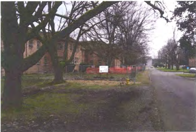
Photo 37: East side of 25th Street NE, north of Mackenzie Hall, looking south
