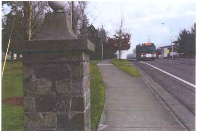
Photo 18: Entry pilaster on north side of NE Center Street
