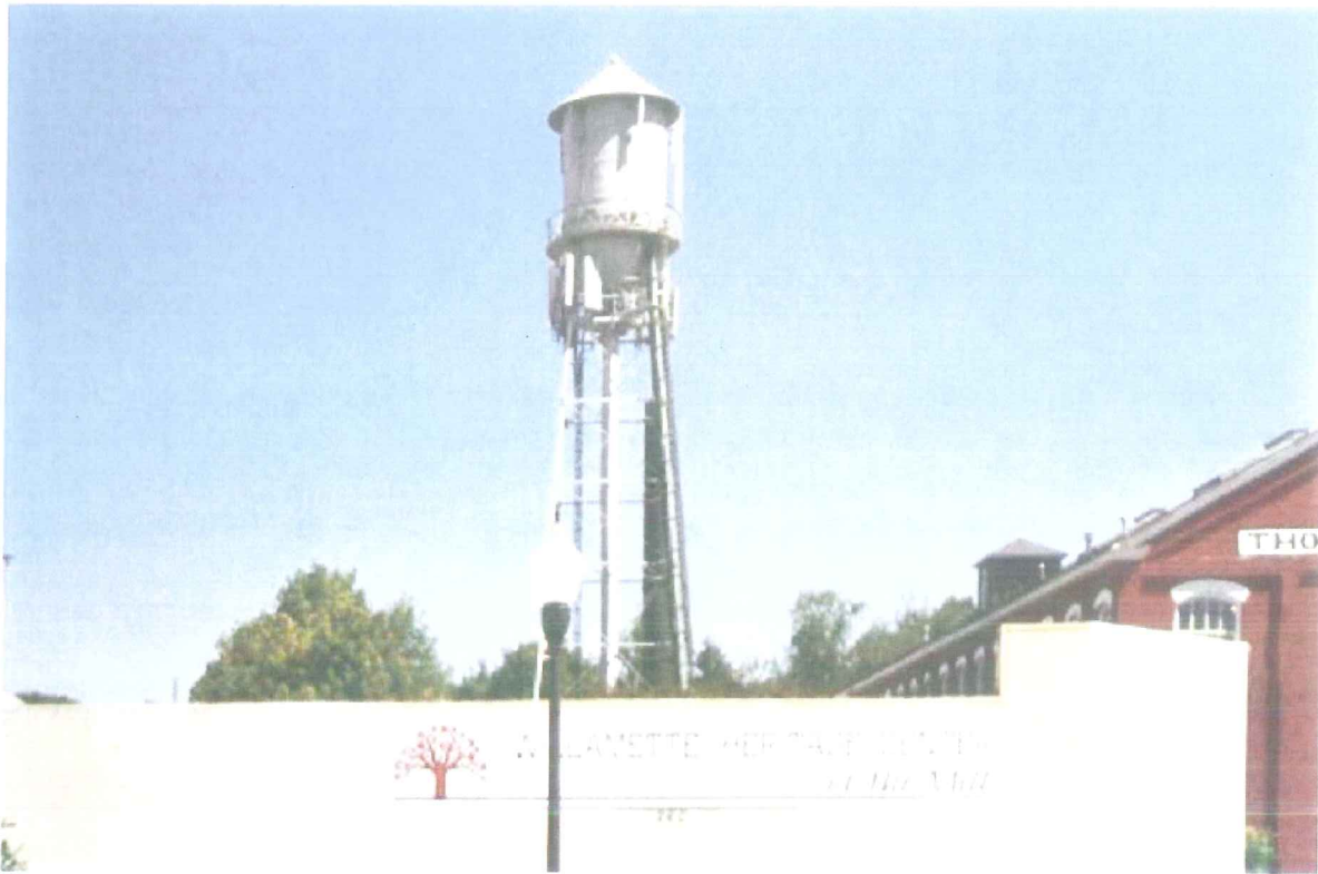
View of SA06 looking East - Existing
