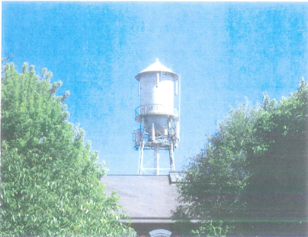
View of SA06 looking North - Existing
