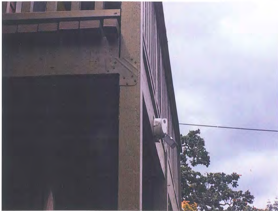
Detail of balcony. Note balcony does not sit on post, but is attached to it.
