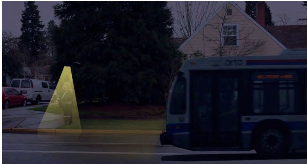
Figures 57 and 58: The two-dim system saves energy by dimming to a lower level of light until a bus patron presses the button to activate the brighter light
