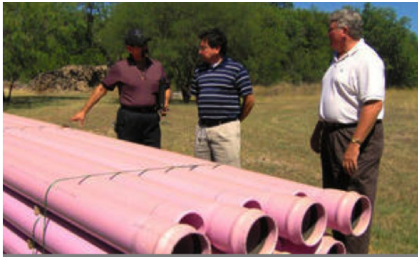
Figure 25: Laying Purple Pipe
