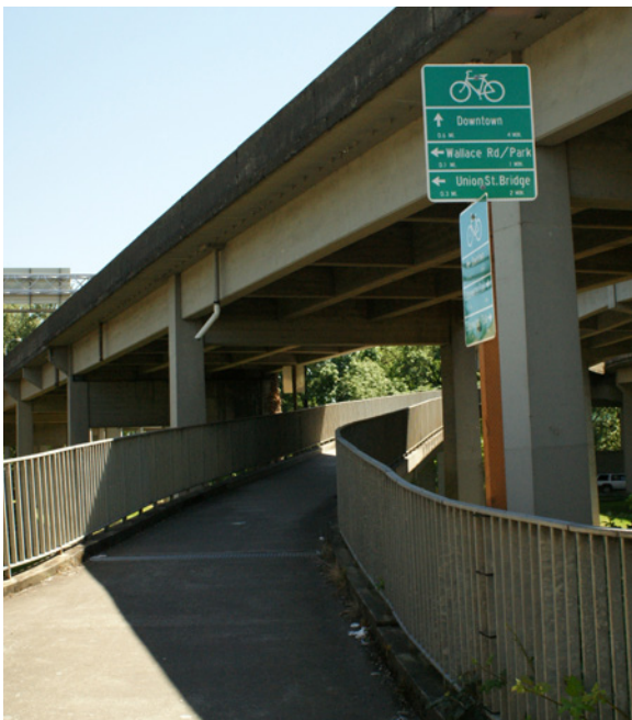
Figure 4: Wayfinding signage assists cyclists with directions in areas where converging bike paths occur and good sight distance is not available.
