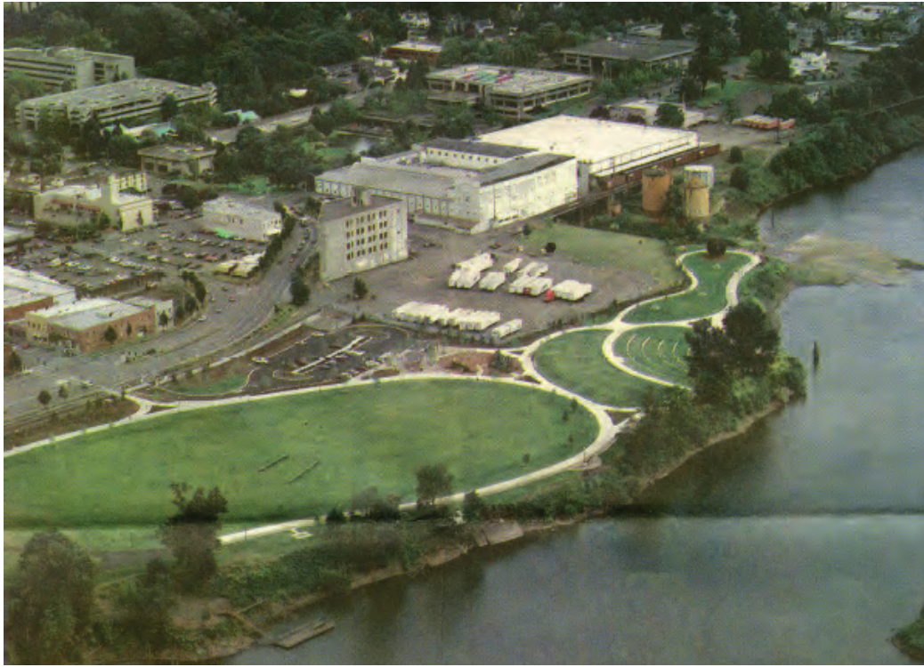
Figure 5: Aerial view of Riverfront Park construction, 1996.
