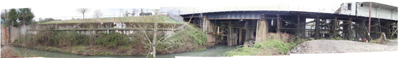
Figure 28: Retaining wall along the north bank of Pringle Creek.
