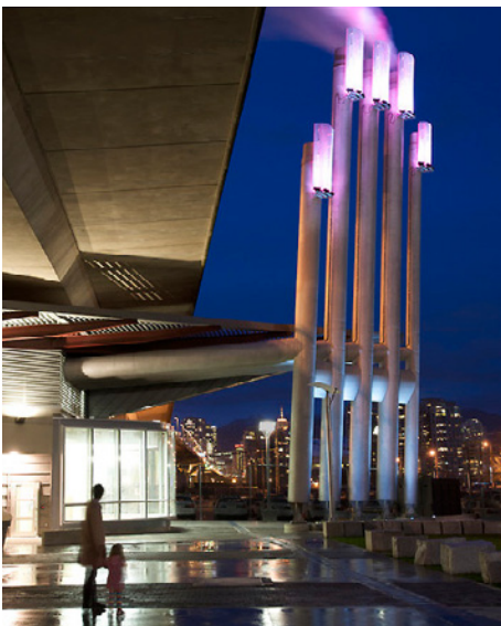
Figure 49: Harvesting the heat of sewer lines to supply the hot water and heating needs of Vancouver, B.C.'s Olympic Village. Source: http://kristophergrunert.tumblr.com/
