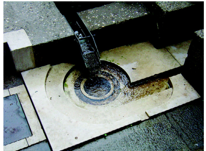
Figures 85 and 86: Exposing natural processes and stormwater infrastructure, Brook Waldman.
