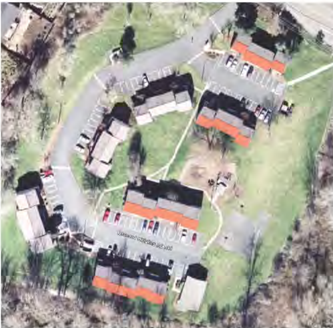
Figure 17: South-facing roof area (orange) at Glen Creek.
