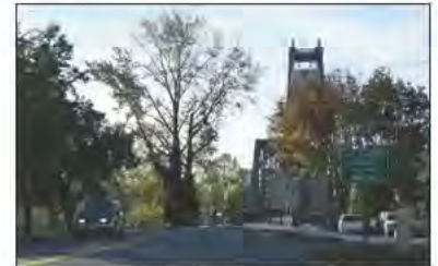
Figure 12: Union Street Railroad Pedestrian and Bicycle Bridge.
