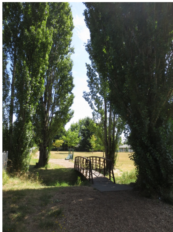
Figure 5. Pedestrian bridge over Claggett Creek
