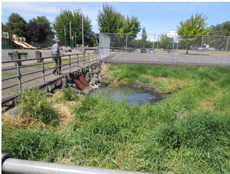
Figure 7. Claggett Creek Outfall
