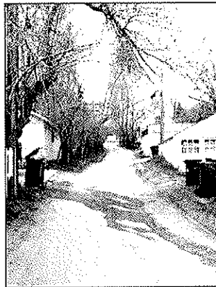
2.3.2 Typical alleys are unpaved and characterized by a variety of small-scale accessory structures and access to parking.
