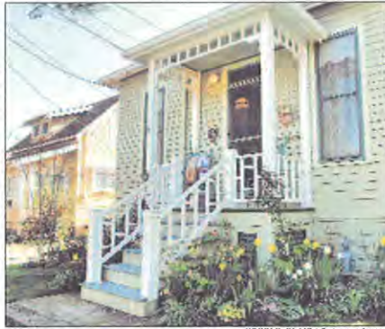
Eleanor Miller lives in the Ethan Graham Cottage in the Court Chemeketa Historic District. She removed the Craftsman style porch and put up the correct Victorian style porch, including railings made of glue and pegs.
