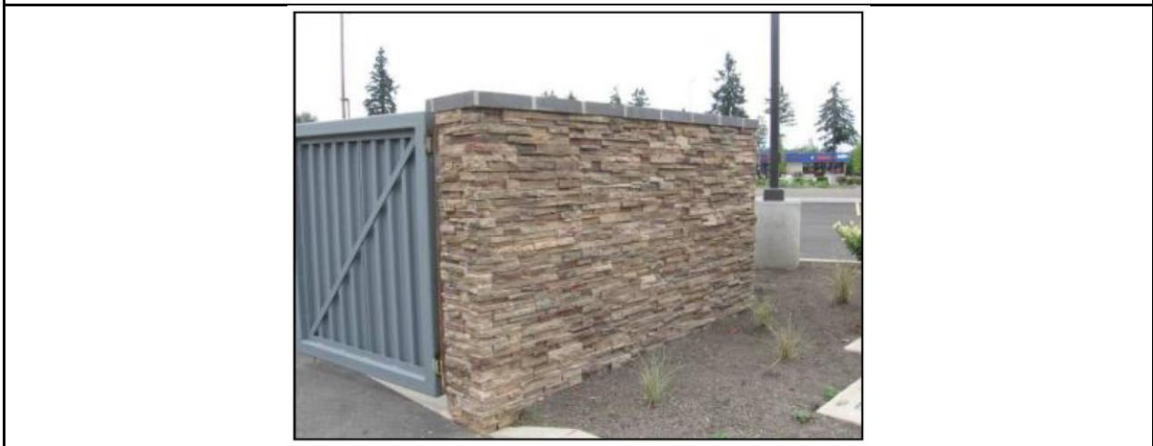
FIGURE 536-9 GROUND-LEVEL MECHANICAL EQUIPMENT
