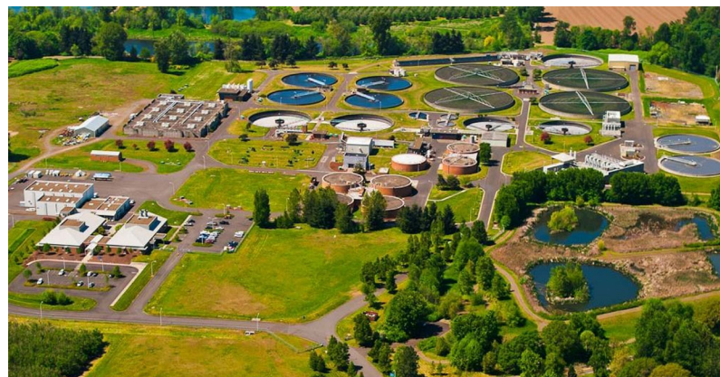
Willow Lake Wastewater Treatment (Source: City of Salem)
