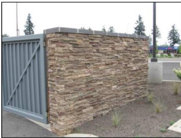
FIGURE 534-8 GROUND-LEVEL MECHANICAL EQUIPMENT
