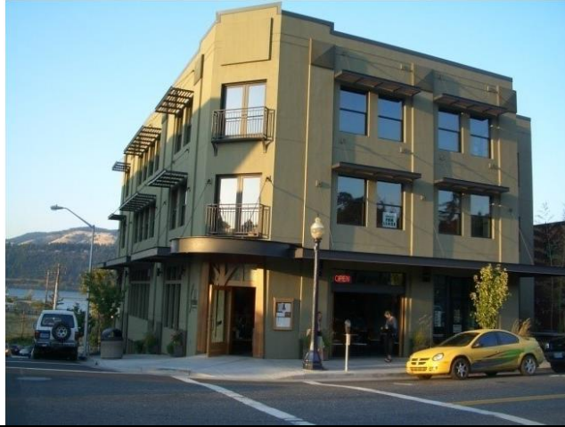
FIGURE 53X-6 ENTRANCE AT BUILDING CORNER
