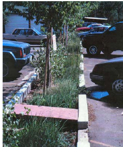
Figure 5. Credits are available to non-SFR customers who maintain a stormwater facility on their property. This rain garden provides both stormwater quantity and stormwater quality benefits.
