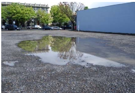
Figure 4. Gravel surfaces that have been subjected to vehicular traffic act like paved surfaces and are considered impervious.
