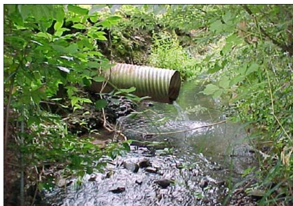
Figure 1. Most stormwater runoff is sent directly into our creeks, lakes, and the Willamette River without treatment. Runoff contains pollutants that can damage the environment. High runoff flows and volumes can erode creek banks and cause flooding.
