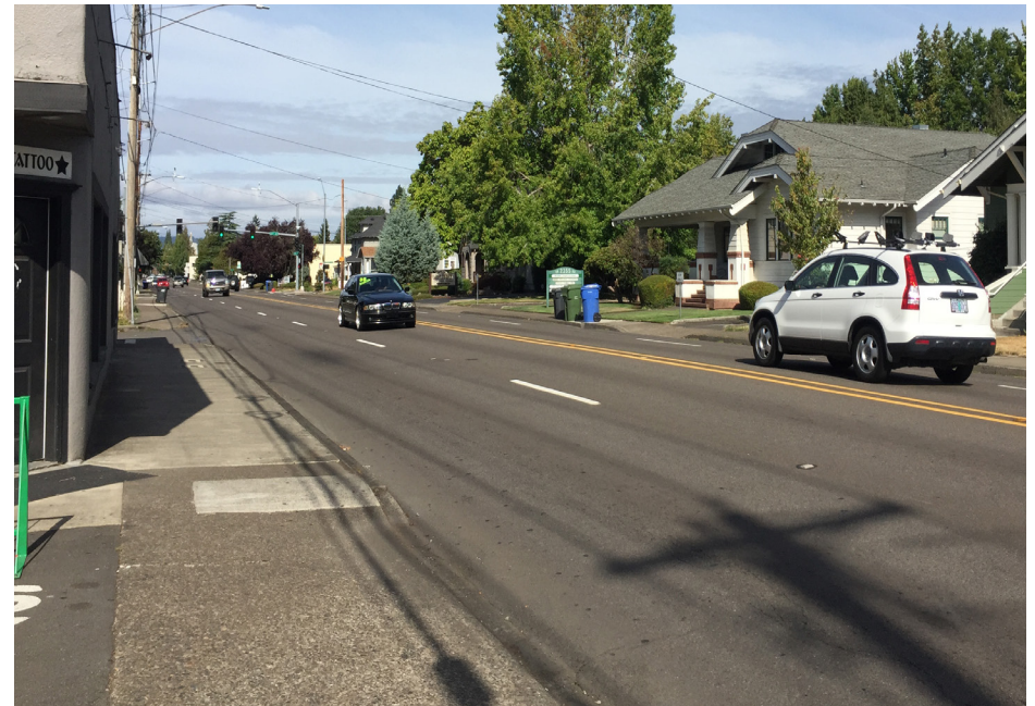
Lack of streetscape features on State Street
