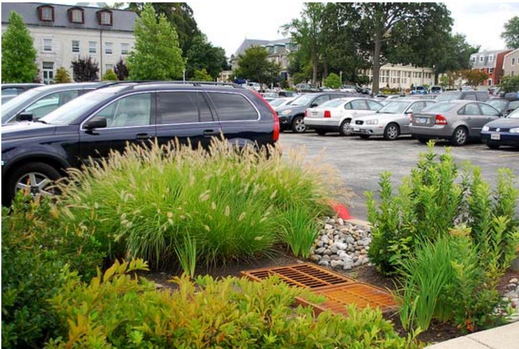
**Figure 9—Example of a Vegetated Bioswale**
