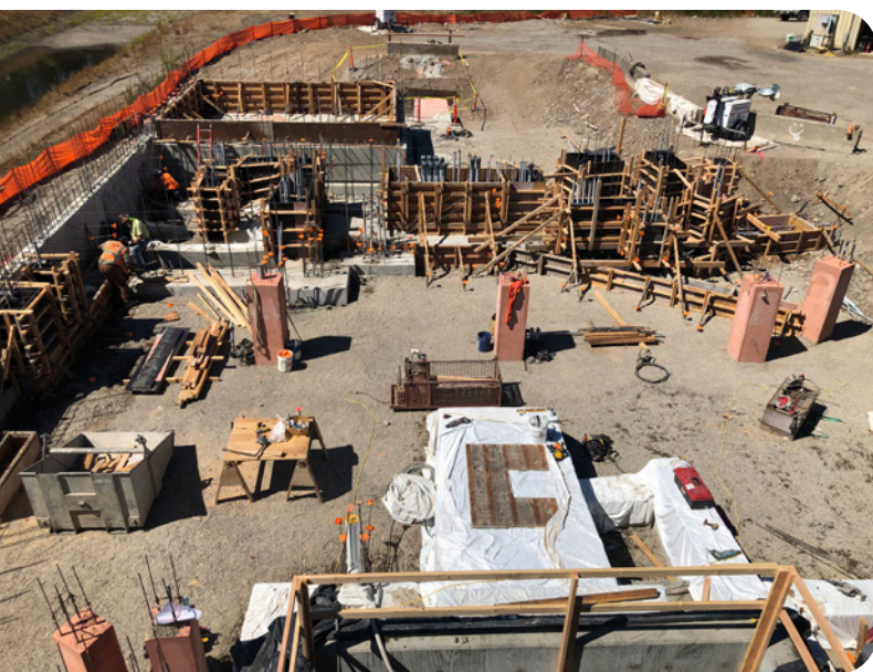
Construction for the new Ozone water treatment
