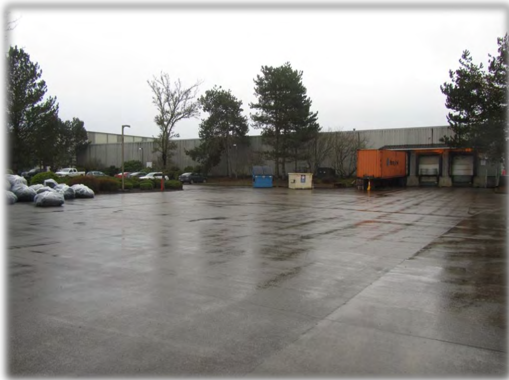
West Coast Washers facility along Turner Road in Area 6. (A12-333)
