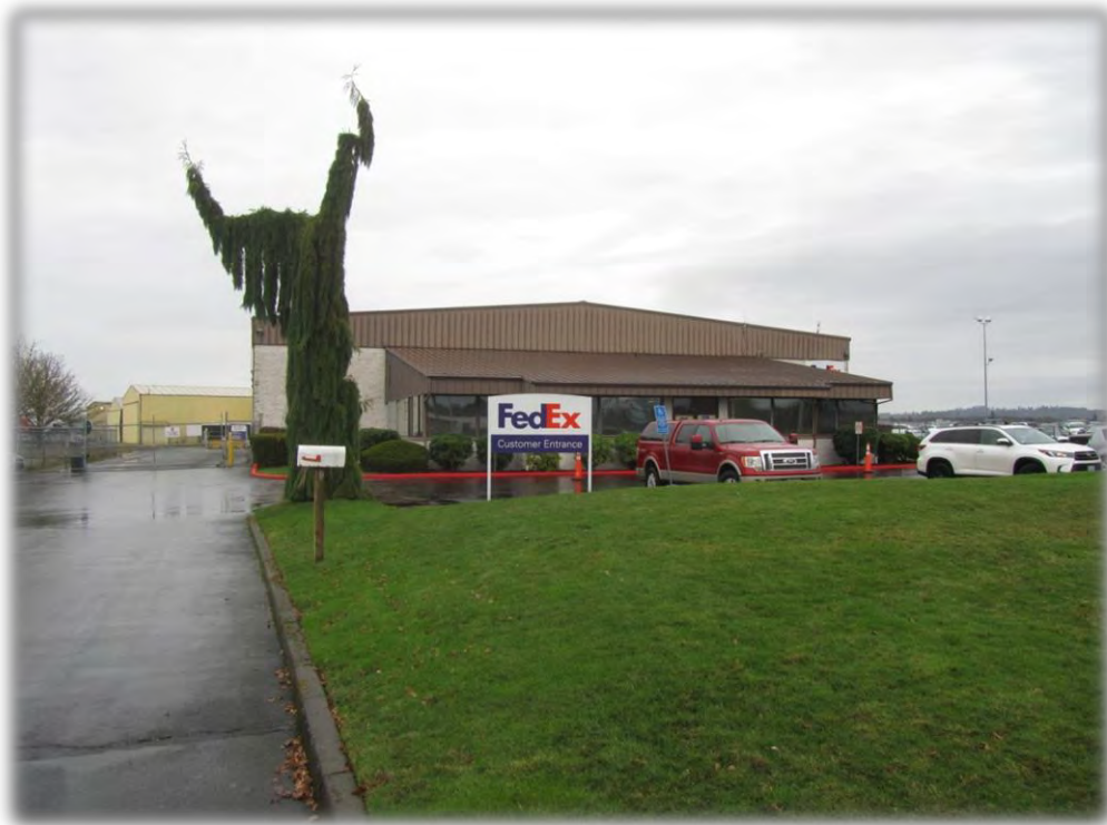
North end of Area 4 showing Fed Ex facility. (A12-344)
