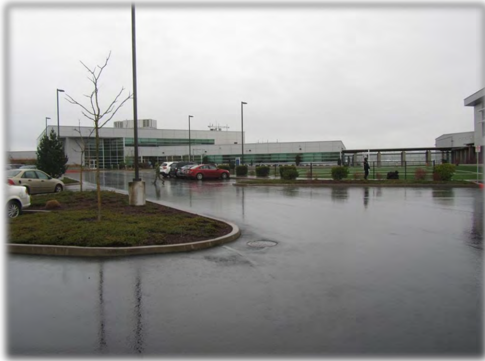
Garmin facility along Turner Road in Area 6. (A12-332)
