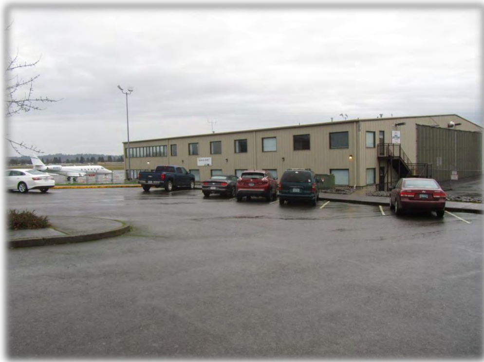
Salem Air Center FBO in south portion of Area 4. (A12-341)
