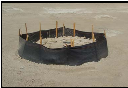
Sediment fence with gravel bags
