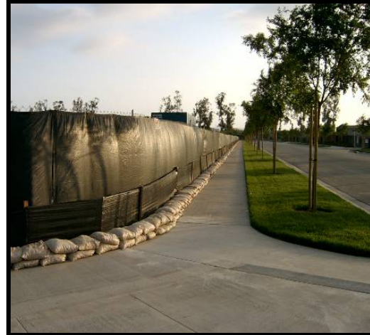
Sediment fence and gravel bags used as perimeter control
