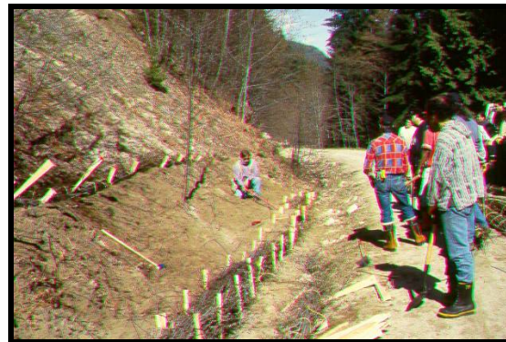
Brush filters being constructed for perimeter control.
