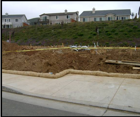
Fiber rolls used as perimeter control
