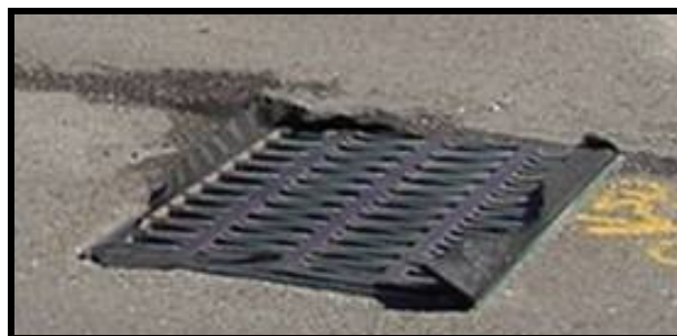
Filter fabric inlet protection
